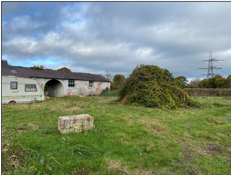
P1 – Site viewed from SE
