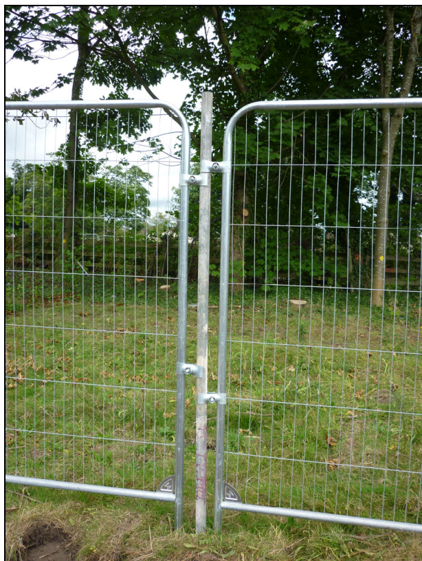
Tree Protective Fencing Specification
