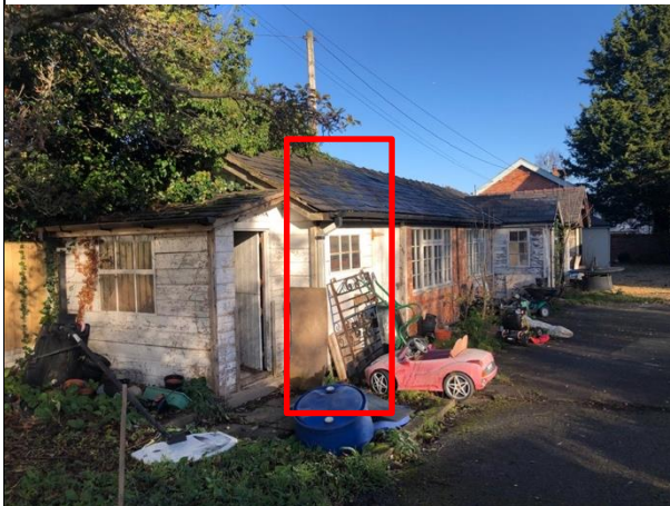
BUILDING FROM SOUTH LOOKING NORTH – SECTION 4 IN RED
