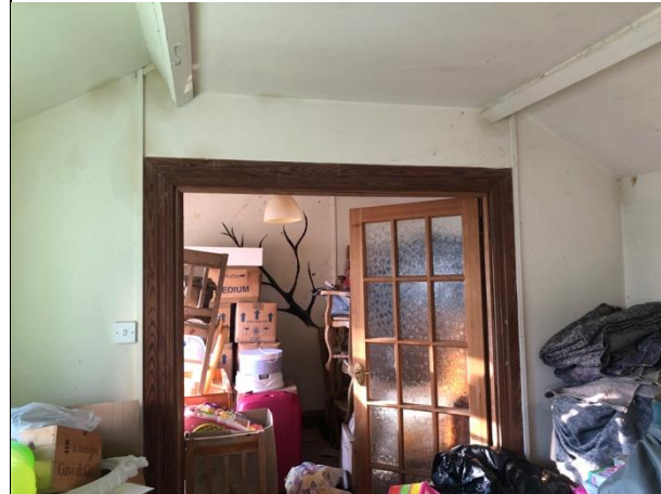
SECTION 3 INTERIOR WITH VAULTED CEILING
