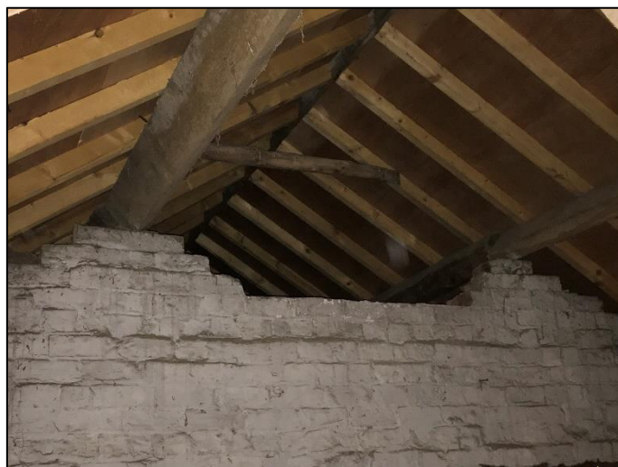
Plate 5. Eastern end of first floor of Barn showing sectioning wall and timber roof frame
