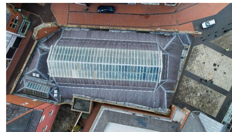
Aerial View 3 of General Market
