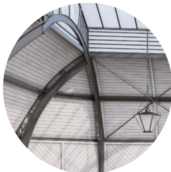
Re-painted structural steel frame
