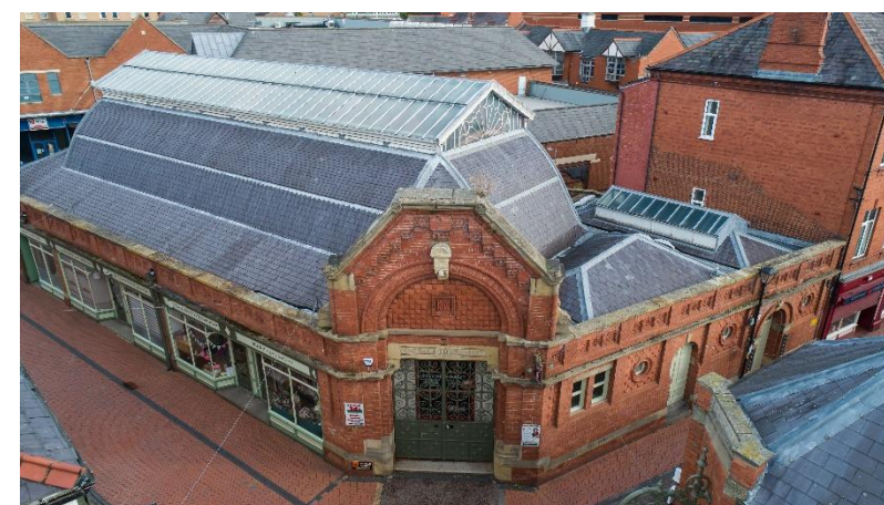
Aerial View 2 of General Market
