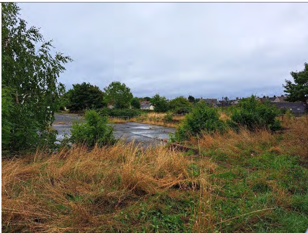
1 – Western part of site, with concrete slab from former community centre building visible
