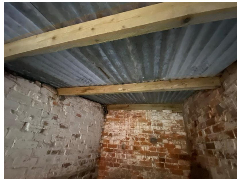
Interior of B2 (pictured above).
