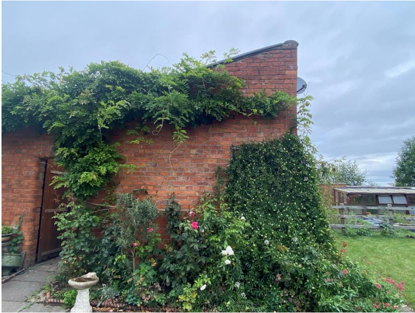
Southern elevation of B1 (pictured above).
