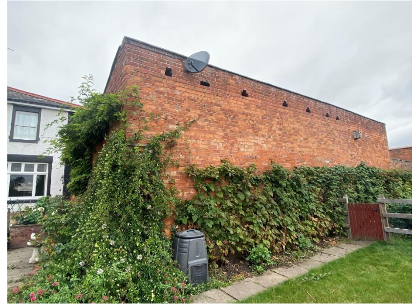
Eastern elevation of B1 (pictured above).
