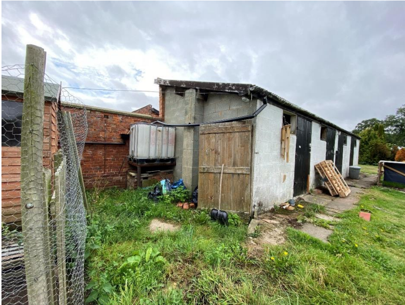
Eastern elevation of B2 (pictured above).
