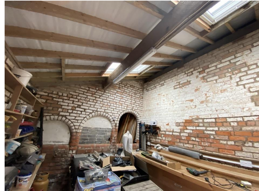
Interior of B1 (pictured above).
