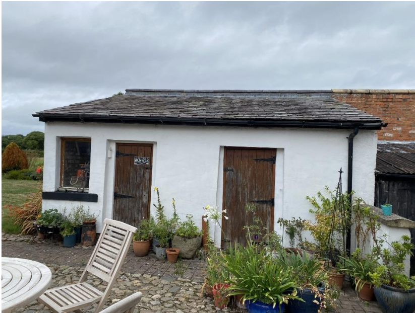
Southern elevation of B2 (pictured above).
