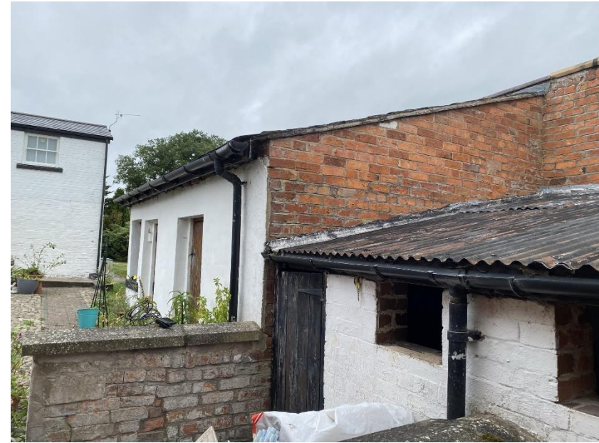
Eastern elevation of B2 (pictured above).
