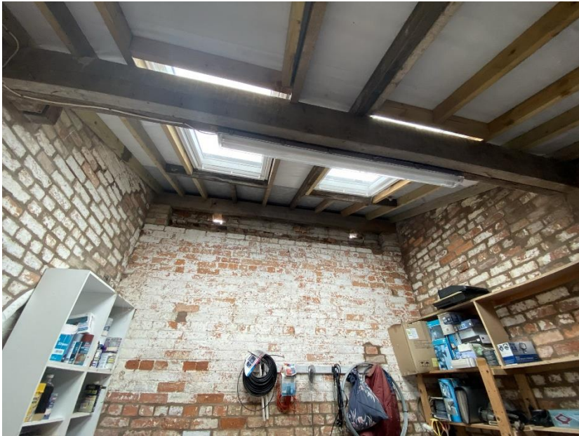
Interior of B1 (pictured above).
