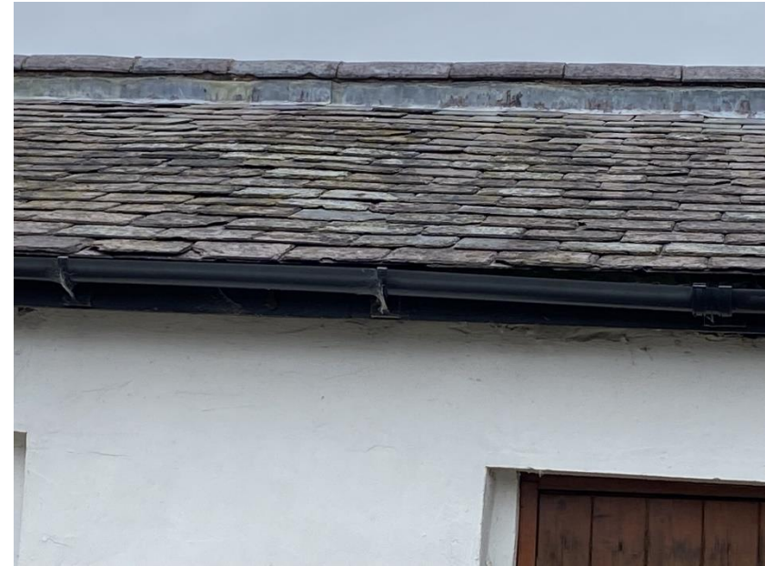
Southern elevation of B2 (pictured above).
