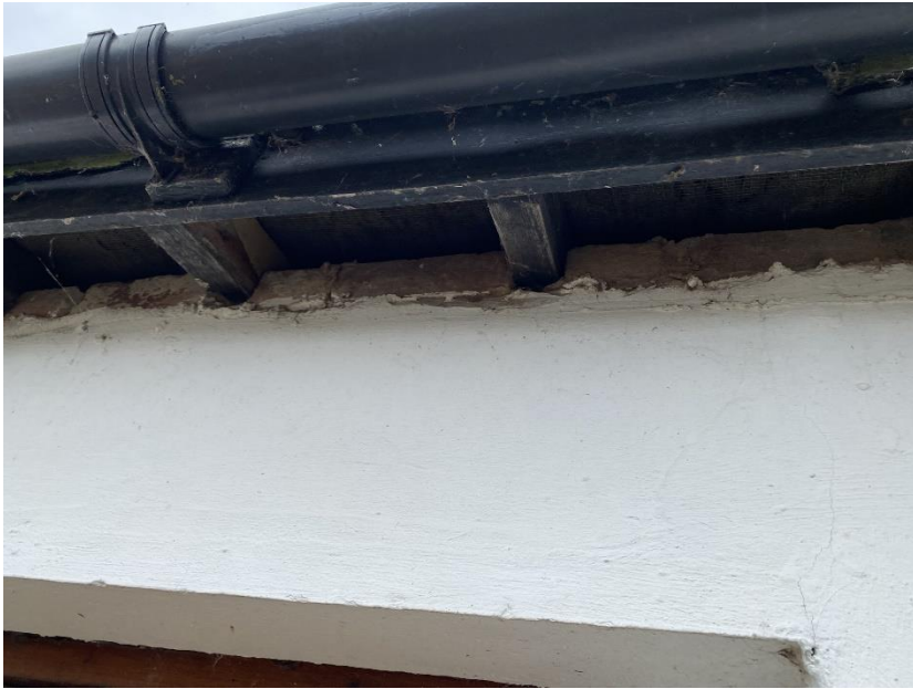
Southern elevation of B2 (pictured above).
