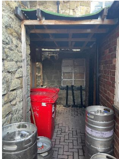
View of the lower rear elevation, within the passage.
