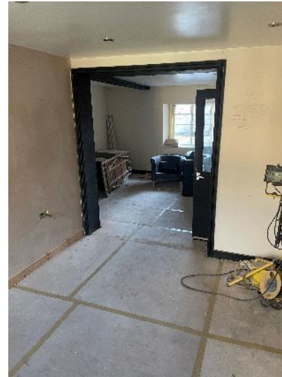
View of the first floor front room viewed from the rear room.
