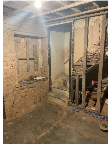
View of the existing staircase – to be retained and repaired where necessary.
