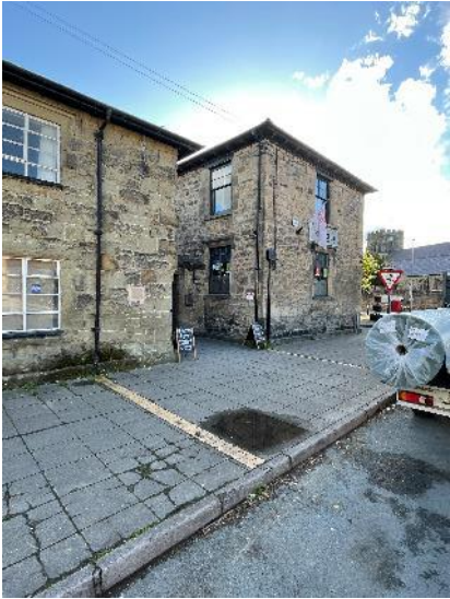
View of the front NW elevation
