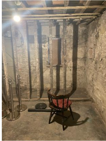
View of the partition to be removed from the ground floor front room.
