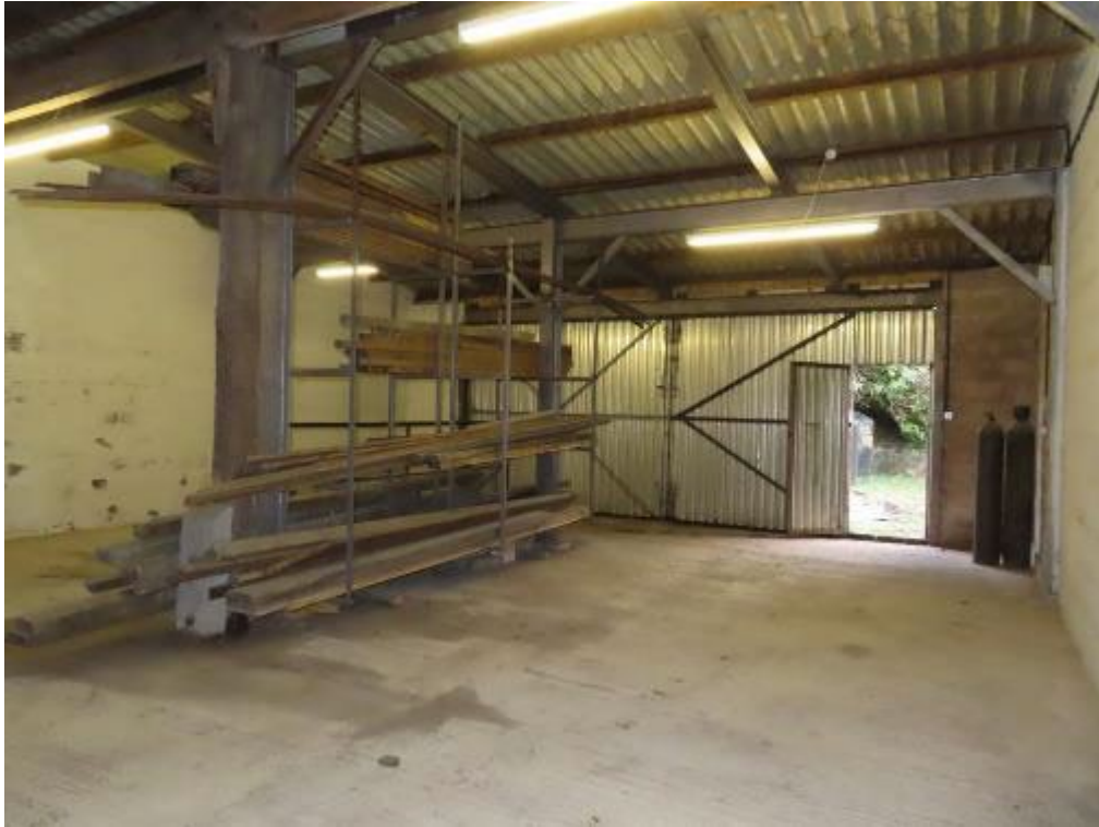
Photograph 14. Interior. View within Section G. Looking northwest from southeast.
