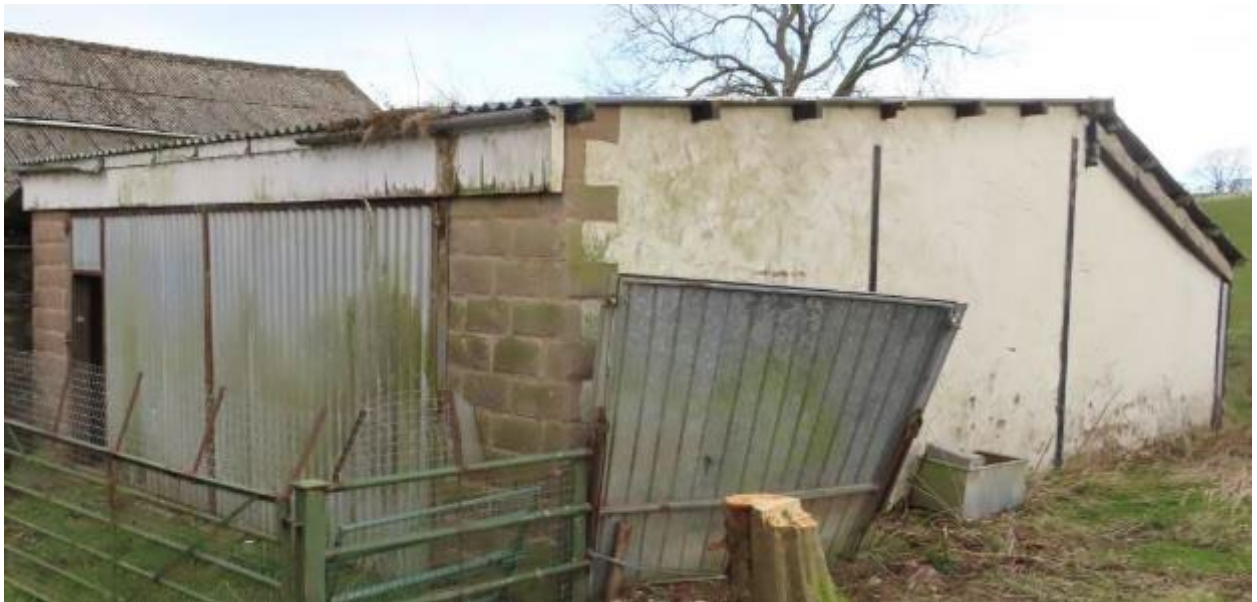
Photograph 13. Exterior. Upper left: part of the Section B and Section D West elevation roof-slopes. Lower left: North elevation of Section G. Right: West elevation of Section G,
