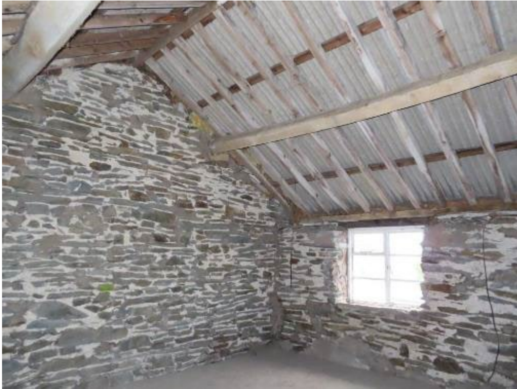
Photograph 9. Interior. View within the Section B north-end first-floor room. Looking northeast from southwest.
