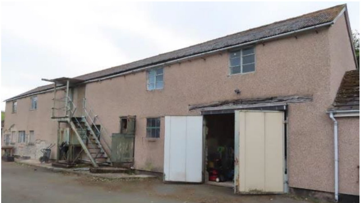
Photograph 4. Exterior. Left, centre and right: East elevation of Section B. Upper far right: part of the North elevation of Section B. Lower far right: part of the East elevation of Section A.
