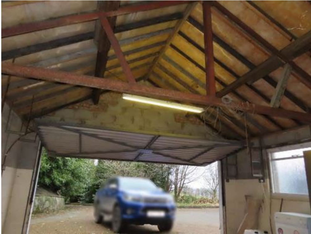
Photograph 3. Interior. View within Section A. Looking north from south.
