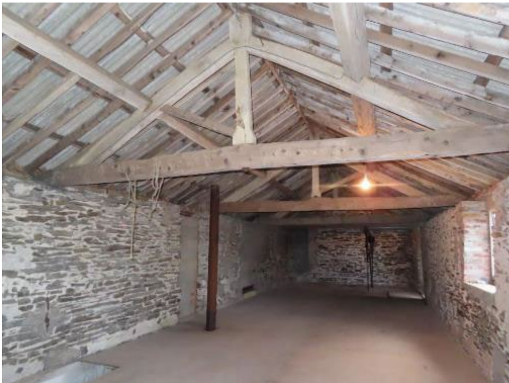
Photograph 10. Interior. View within the Section B central and south-end first-floor room. Looking northwest from southeast.
