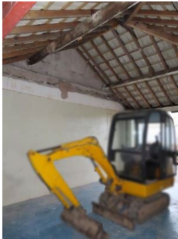
Photograph 12. Interior. View within Section E. Looking northeast from southwest.
