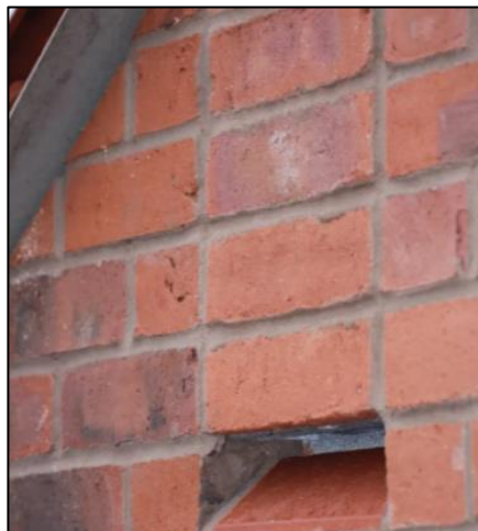
Bat box built into external wall.
