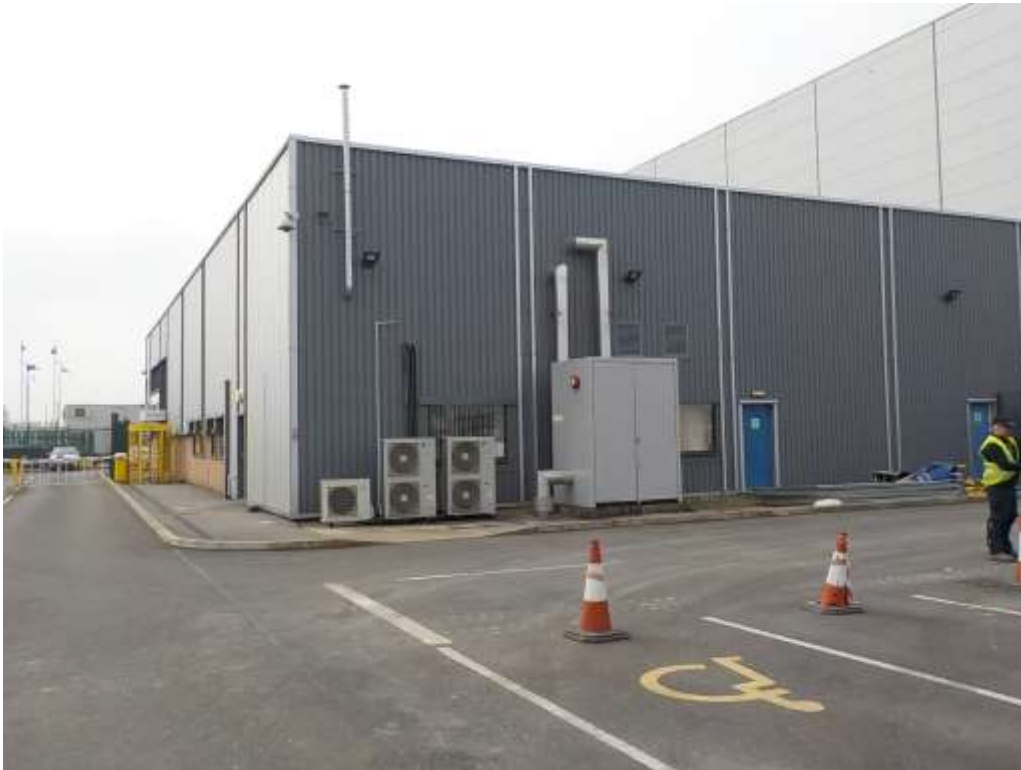
Building proposed for demolition
