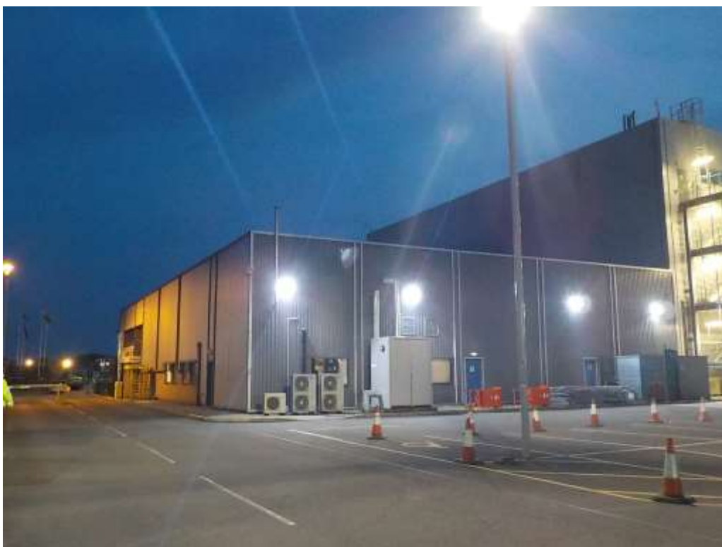
High levels of lighting around the building during the hours of darkness
