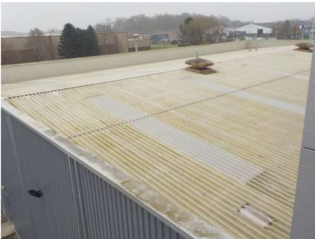
Roof of the building, showing Perspex panels
