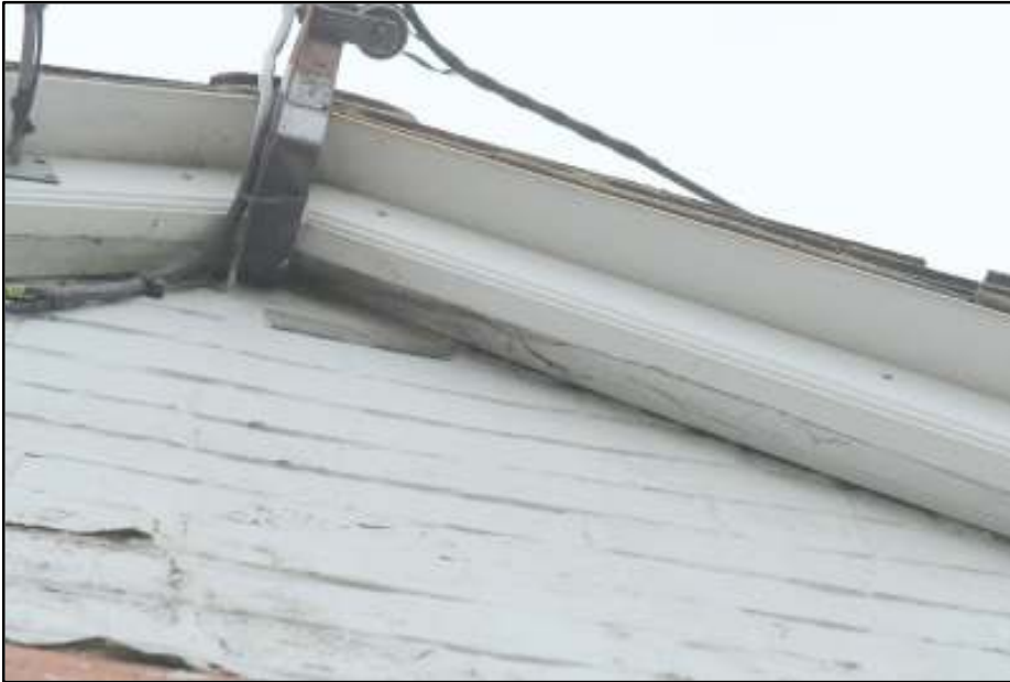
Sealed behind the gable fascia boards
