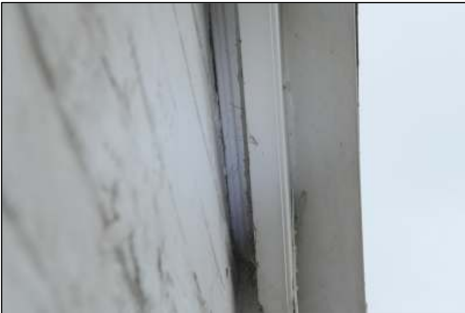
Sealed behind the gable fascia boards
