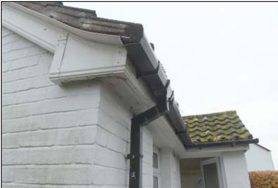
UPVC soffits are well sealed with no gaps
