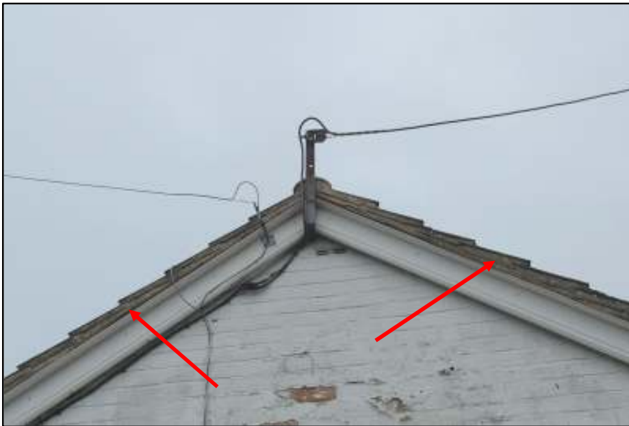
Gables are well sealed with intact mortar below the edge of the tiles
