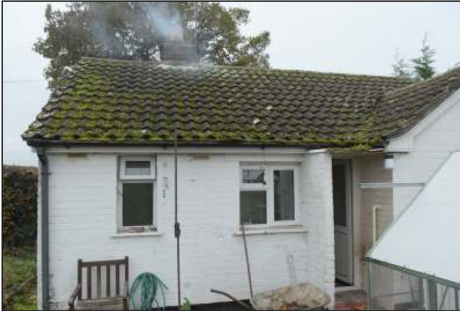
UPVC soffits are well sealed with no gaps
