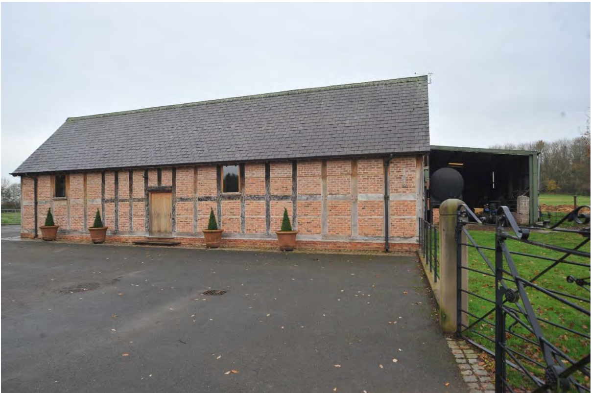
Pl.8: The Grade II listed timber-framed range to the east of the house.
