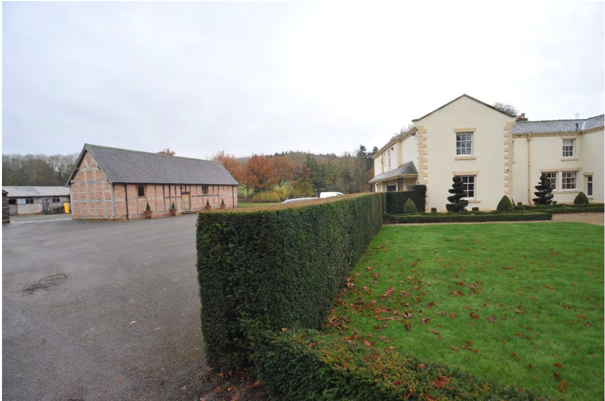
Pl.9: The relationship between the house and listed barn, viewed from the north.
