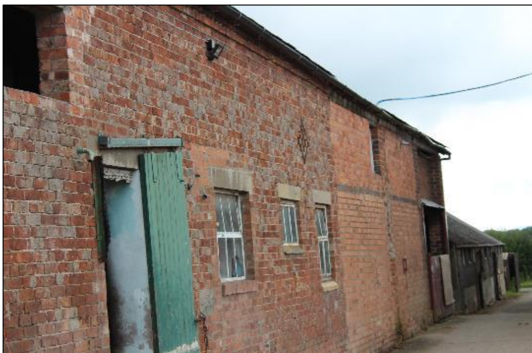
Plate 1 - Barn, north-west elevation looking south-west
