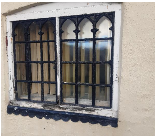
Existing cast iron window casements intersecting round heads
