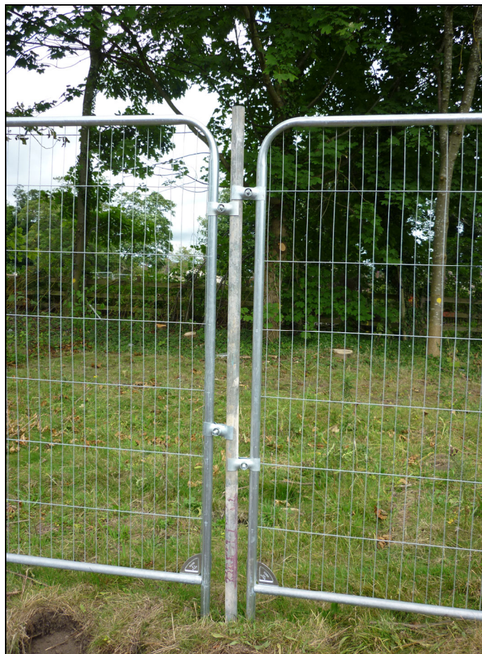
Tree Protective Fencing Specification
