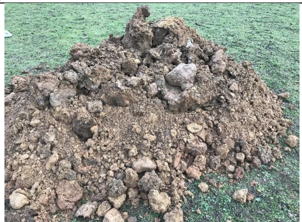
Soakaway Pit 04: Excavation spoil.
