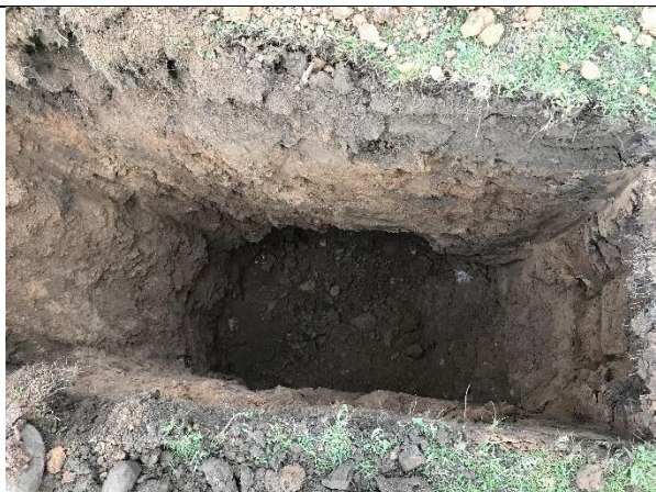
Soakaway Pit 05: Internal view of excavation.
