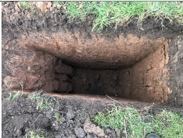
Soakaway Pit 03: Internal view of excavation.
