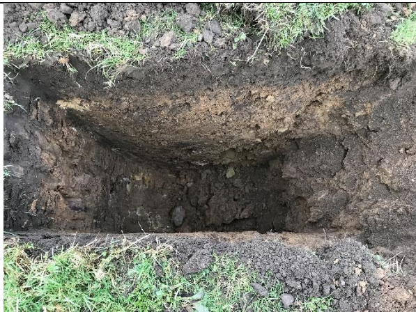
Soakaway Pit 02: Internal view of excavation.
