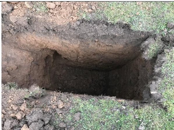
Soakaway Pit 01: Internal view of excavation.
