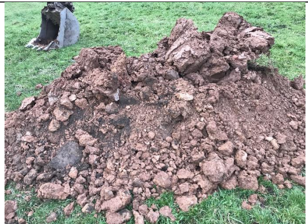
Soakaway Pit 03: Excavation spoil.
