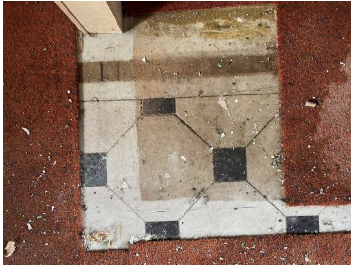
Plate 16 - Floor tiles exposed in G1
