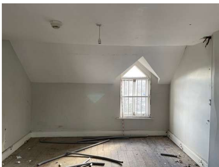
Plate 41 - Southeastern wall of S2
