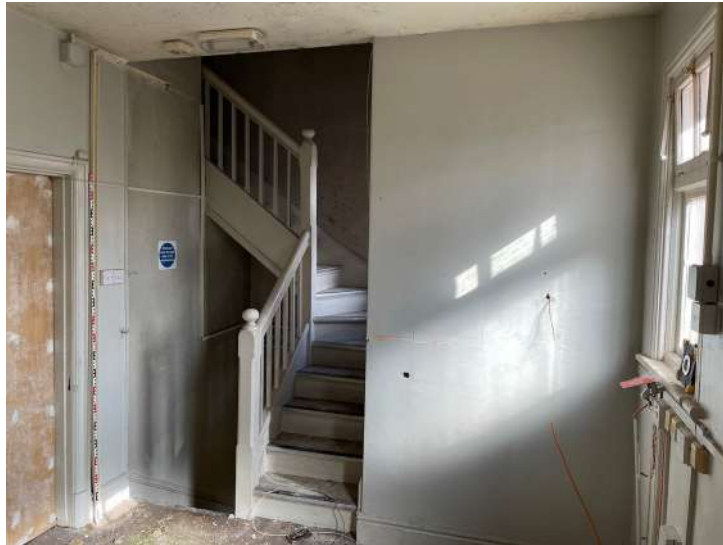
Plate 22 - Room G3, looking north
