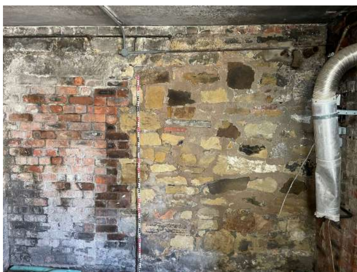
Plate 49 - Northwest wall of L2
