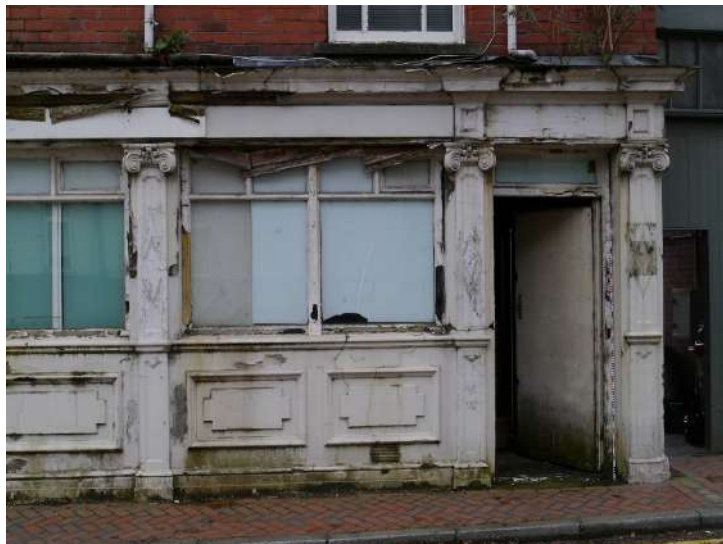
Plate 5 - Southern end of northwestern elevation
