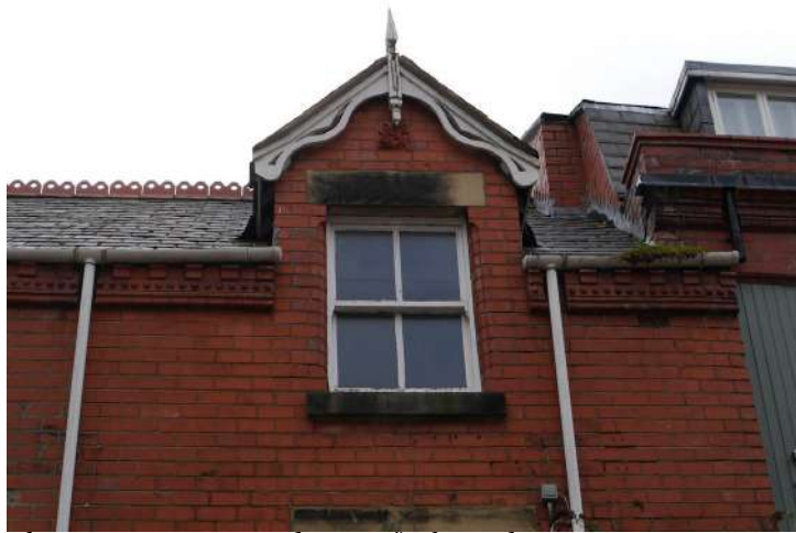
Plate 2 - Dormer window, roof tiles and terracotta cornice
