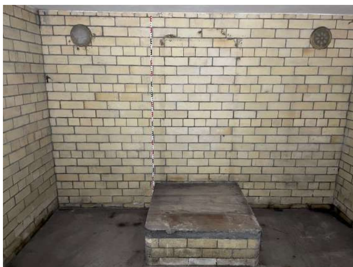
Plate 54 - Brick platform and ghosting of safe
