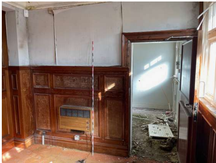
Plate 19 - Northeast wall of G2
