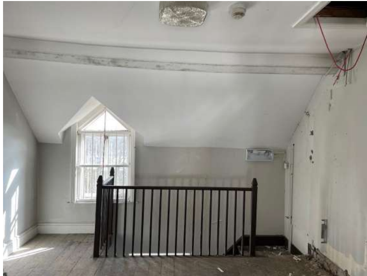
Plate 36 - Southeastern wall of S1
