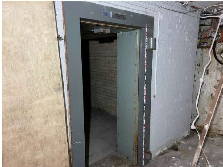
Plate 51 - Vault access in L3
