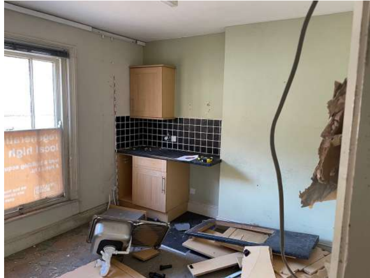
Plate 30 - Room F2 looking north
