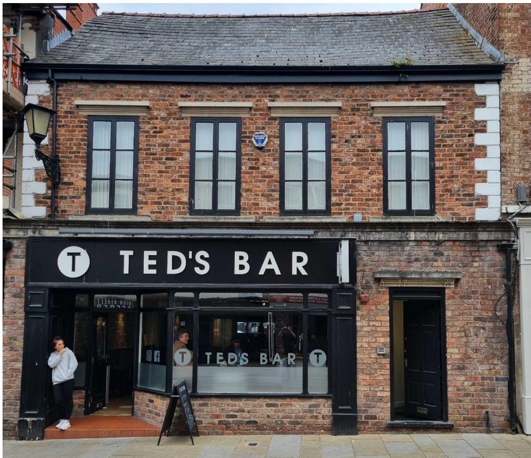
Front View of 36 High Street
