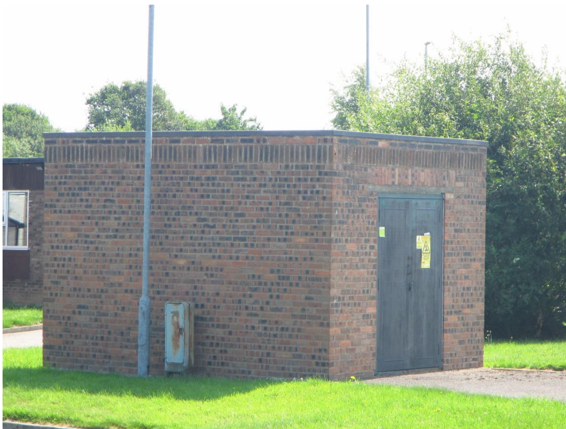
Photograph 25 – Western and southern aspect of Building 10.
