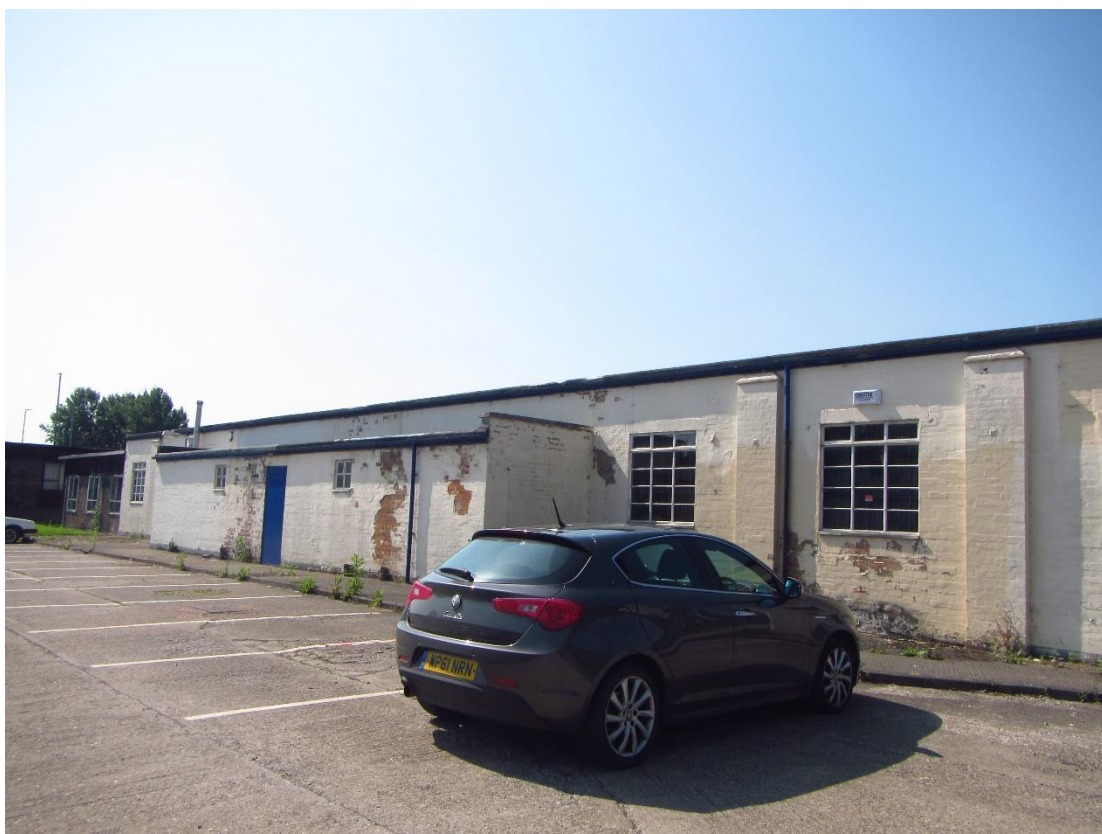
Photograph 7 – Northern aspect of Building 2.
