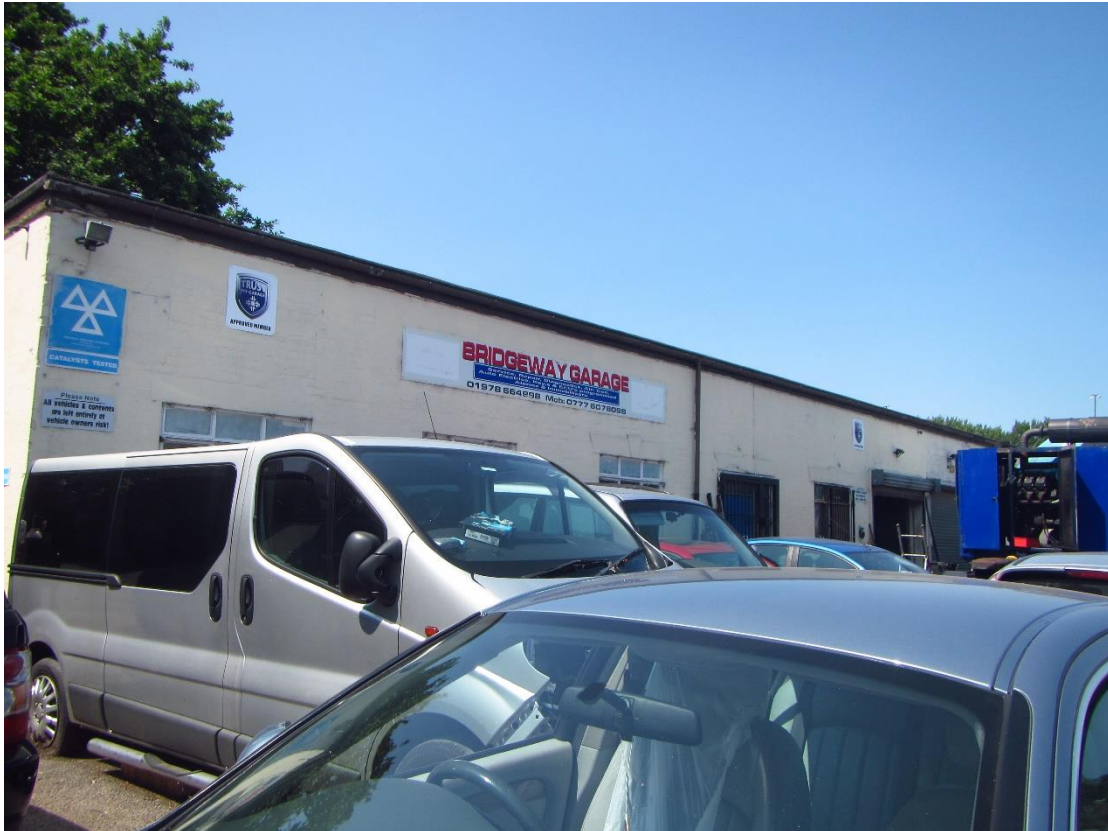
Photograph 24 – Northern aspect of Building 9.
