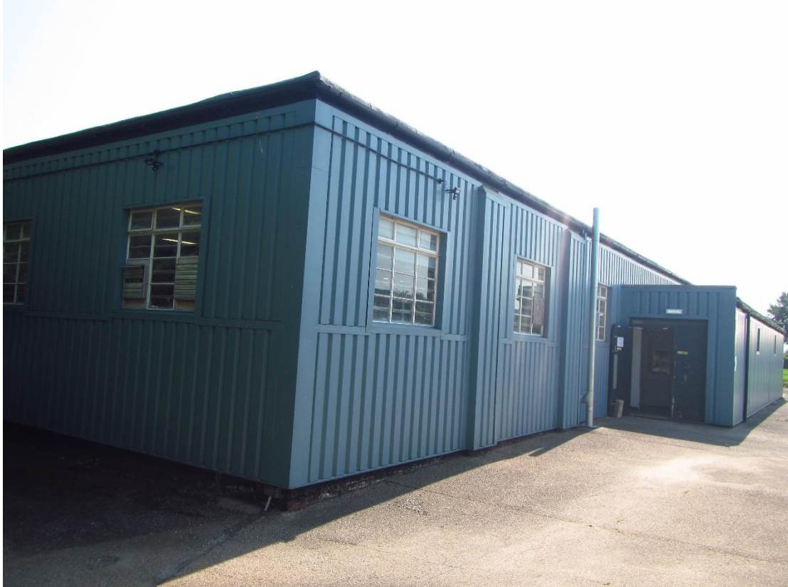
Photograph 12 – Western and southern aspect of Building 3.
