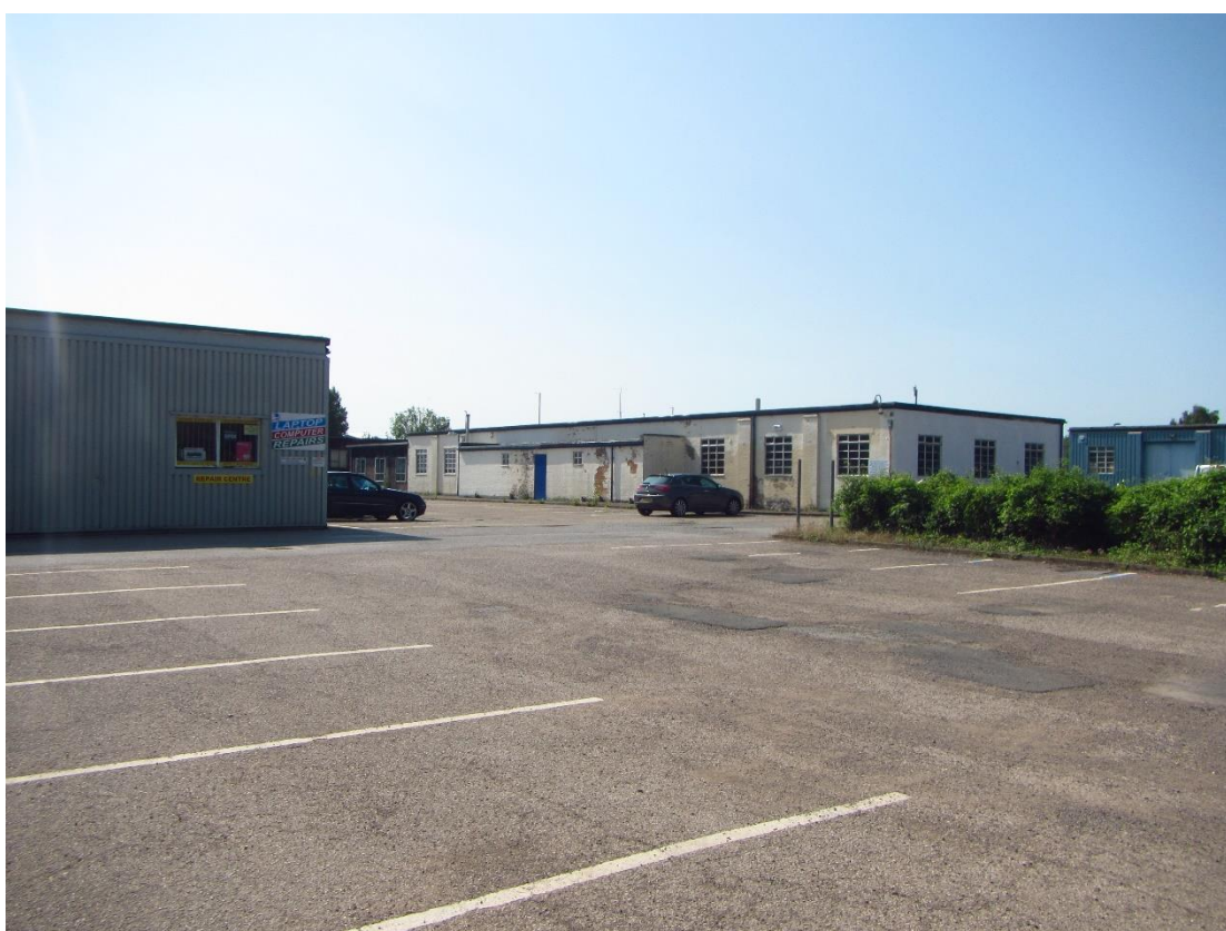
Photograph 8 – Northern and western aspect of Building 2.
