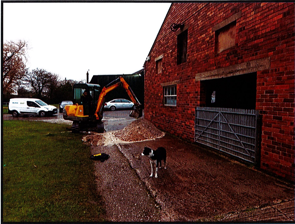
Trial Pit Location
