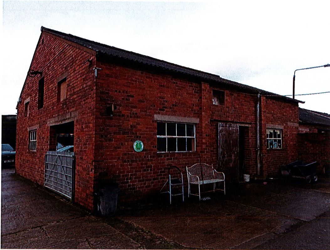
Photograph 3 Other side of Barn
