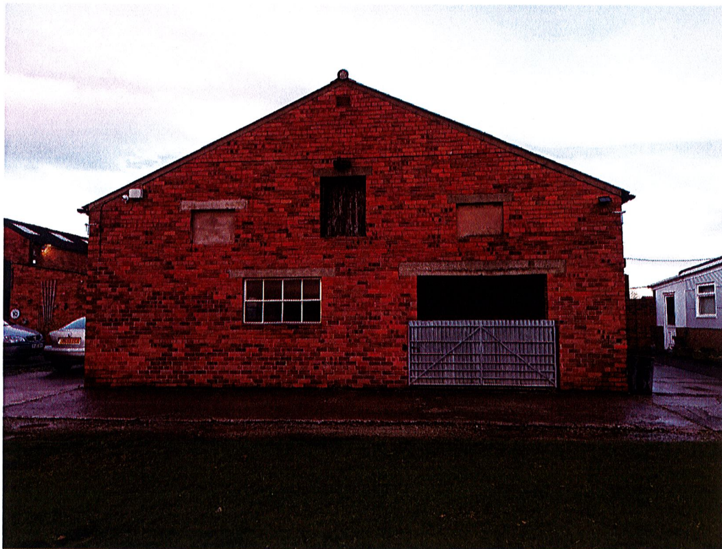
Photograph 4 Front of barn
