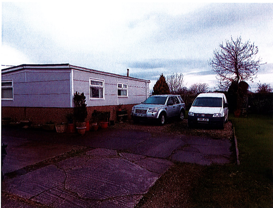
Photograph 6 Existing temporary accommodation
