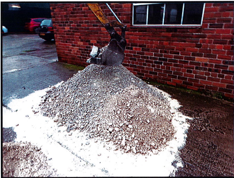
Spoil arisings comprising sub base material
