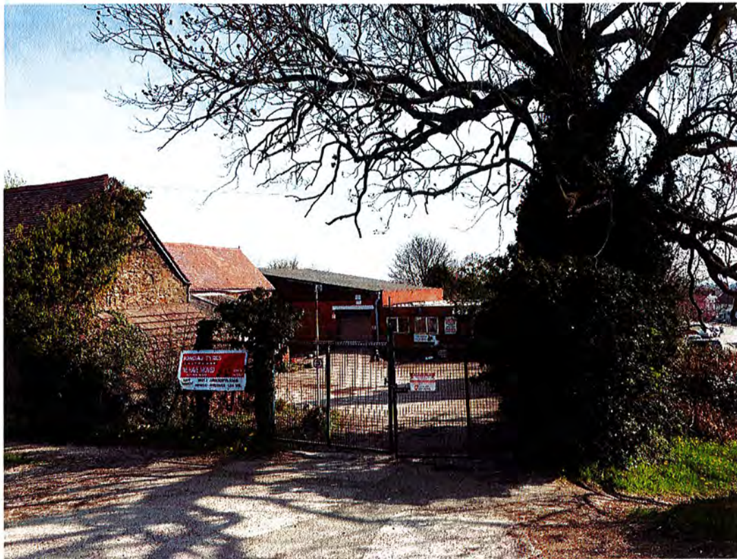
Photograph 1 – Site entrance from Ruabon Road, showing existing buildings
