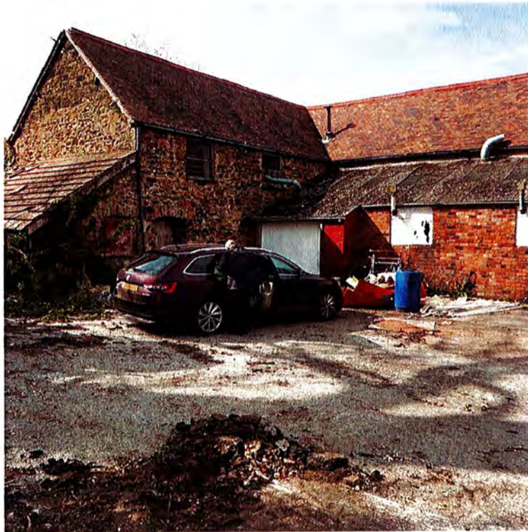
Photograph 3- Facing west showing existing masonry building.
