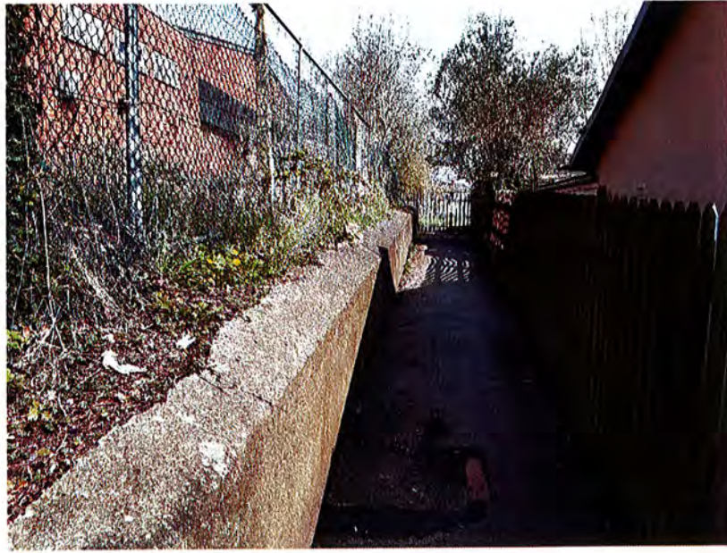
Photograph 9- Showing Retaining wall on eastern site boundary.
