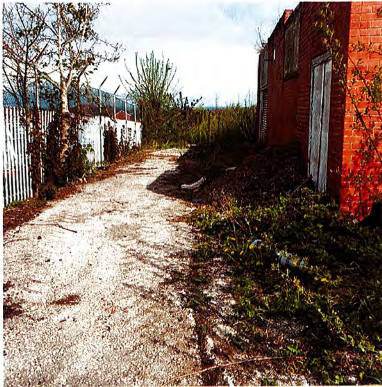
Photograph 11- Facing east showing boundary with school to the north and back of the industrial unit.
