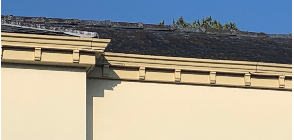
Photograph 3. Example damage to soffit boxes
