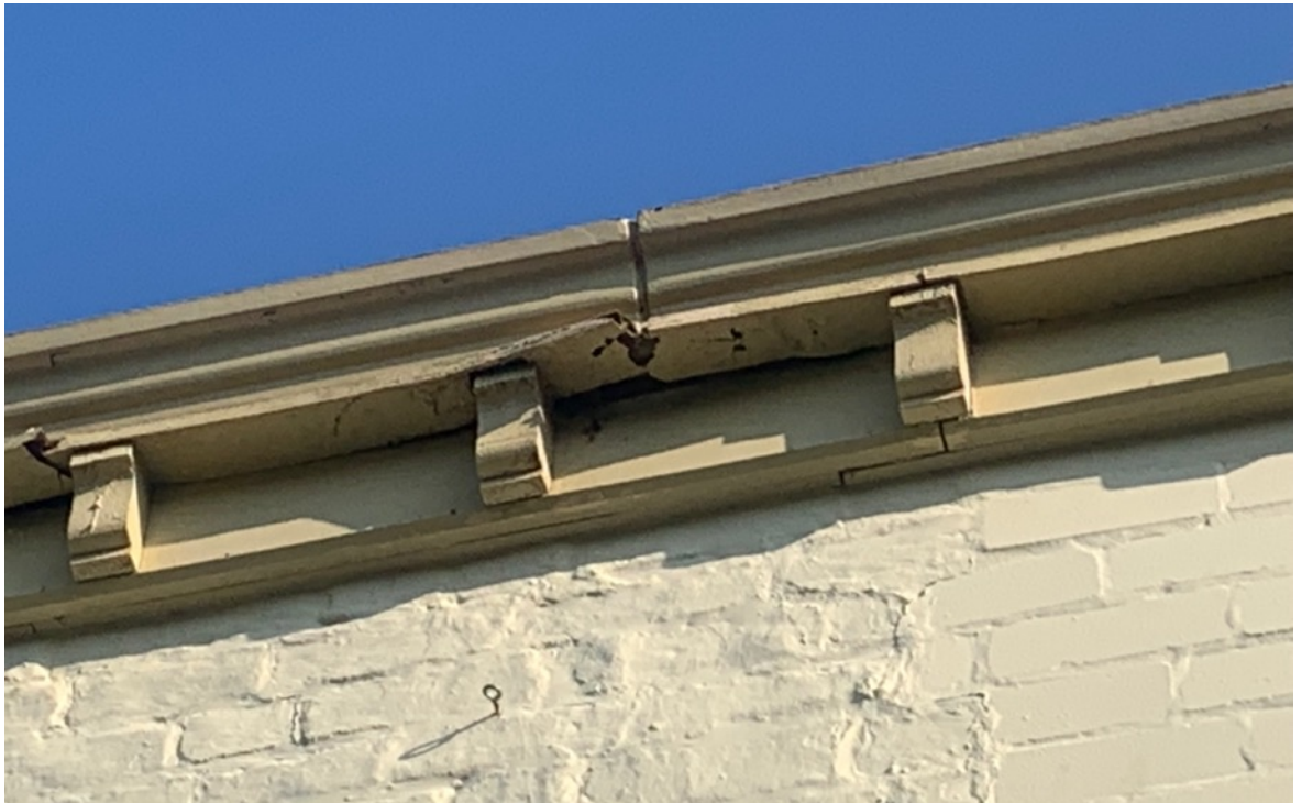
Photograph 3. Example damage to soffit boxes
