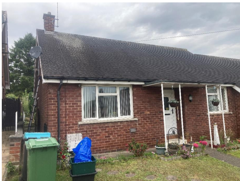
A1.1 Plate 1 – Shows the front elevation, facing towards the East
