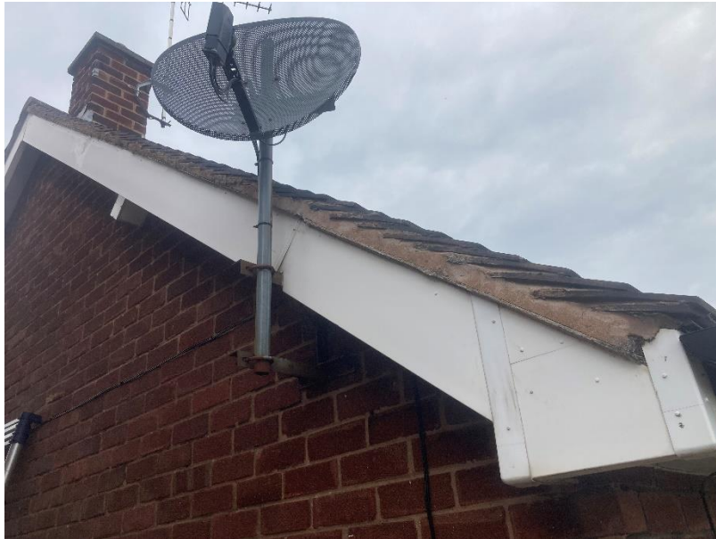
A1.4 Plate 4 – Showing the very well sealed soffit box
