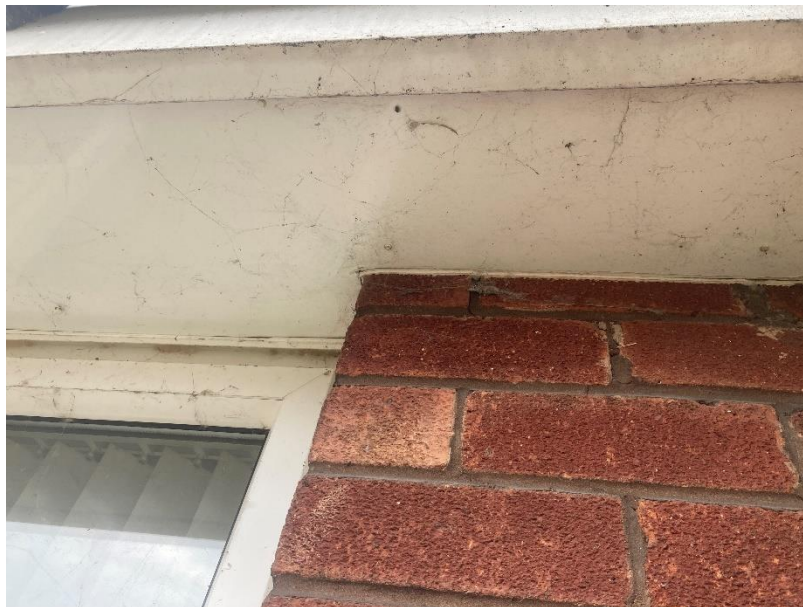
A1.4 Plate 4 – Showing the very well sealed soffit box
