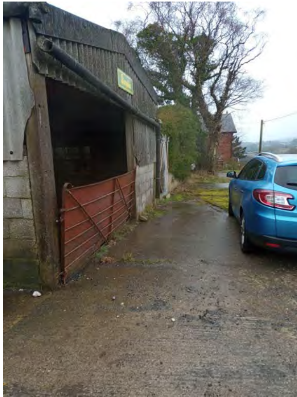
Photo 5: View along the western boundary of the Site.
