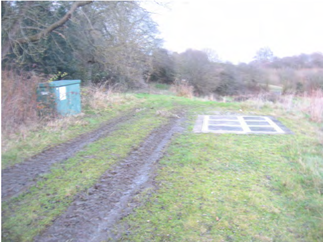
Photo 5 – Underground tanks relating Welsh Water
