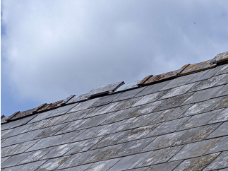
photograph showing ridge tiles raised to allow bat access as per ecological survey.
