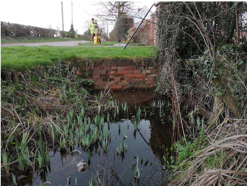
Photograph of the upstream face of blocked Culvert structure Culv_1.16 (NGR 346160 335340):
