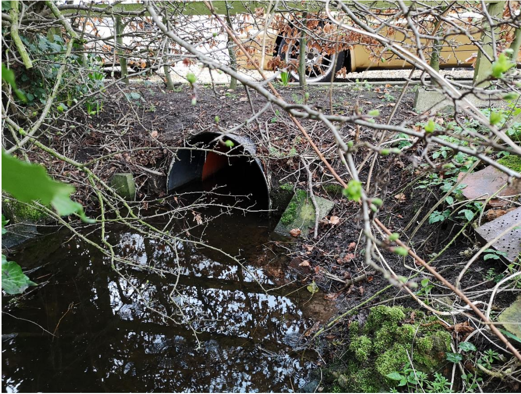
Photograph of the upstream face of blocked Culvert structure Culv_1.16 (NGR 346160 335340):
