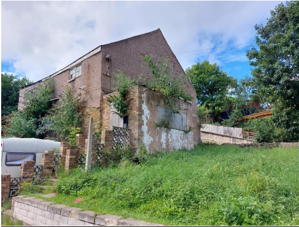
Side elevation of Chapel Farmhouse
