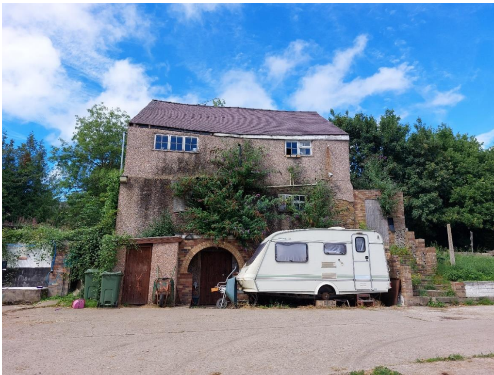
Front elevation of Chapel Farmhouse
