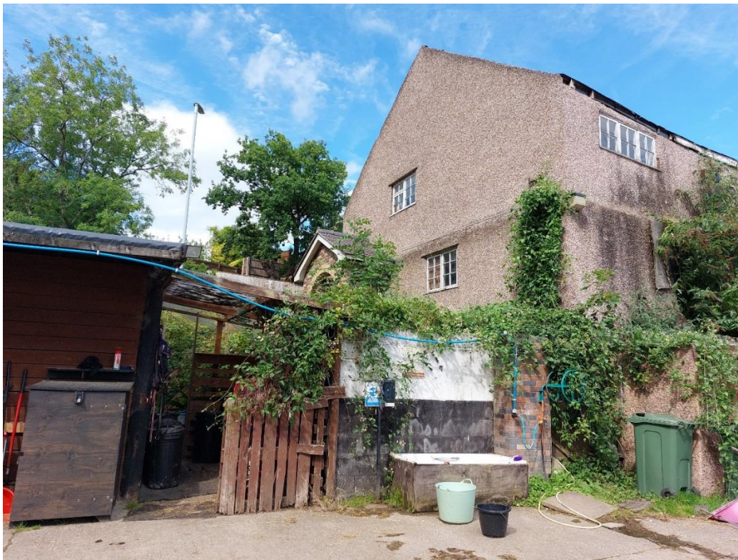
Side Elevation of Chapel Farmhouse
