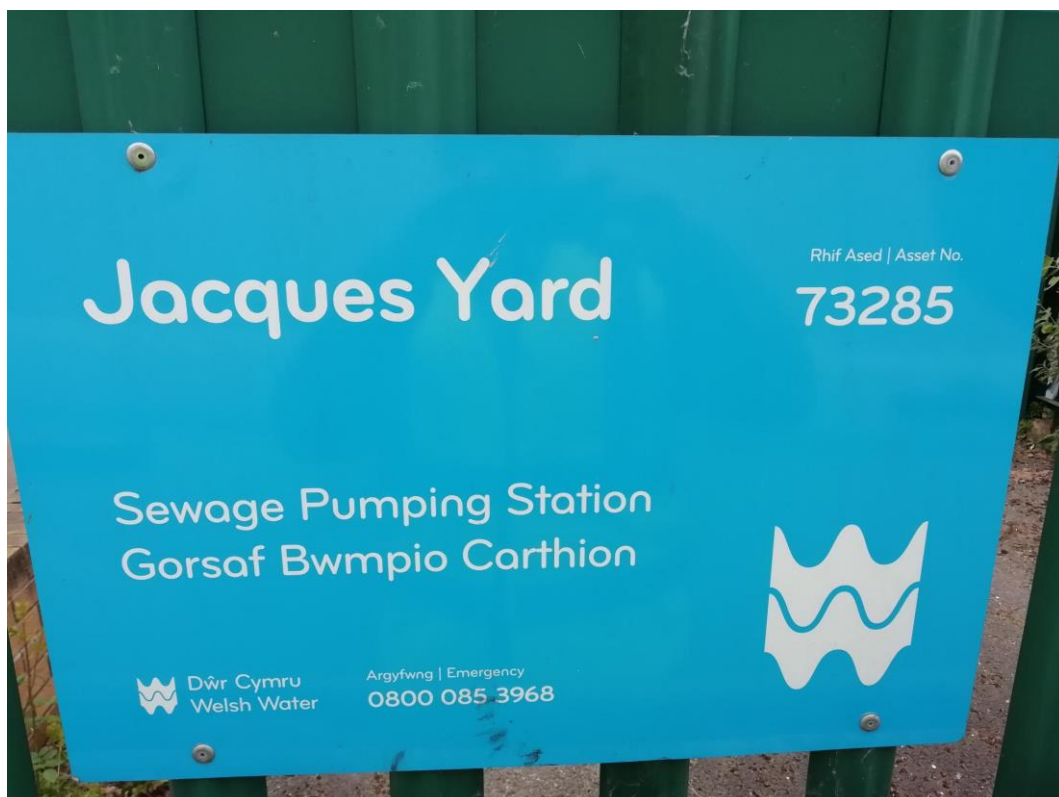
Figure 3-3: Sewage Pumping Station – Picture 3
