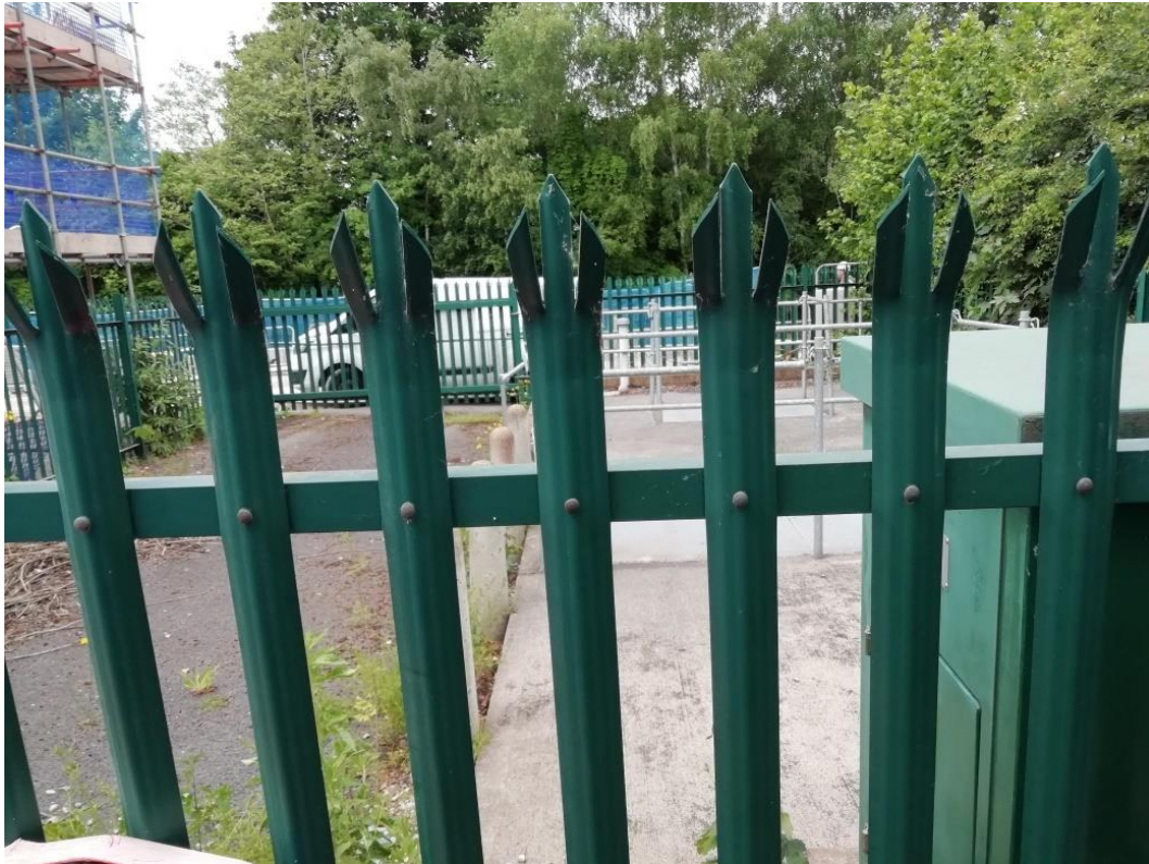
Figure 3-2: Sewage Pumping Station – Picture 2
