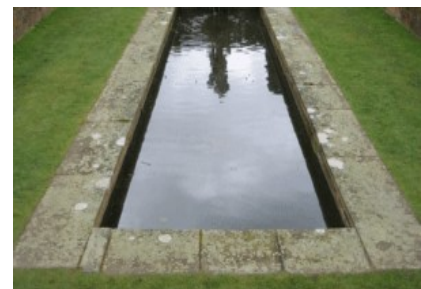
Simple line of stone coping stone to pool using York stone to match the path.
