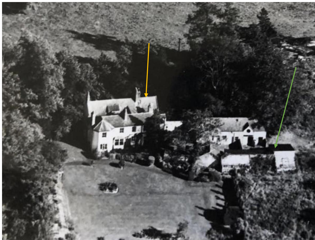
Fig 5. An undated aerial photograph of the rear of The Lodge, which appears to pre-date 1948. This shows the lost bay (arrowed yellow). The outbuildings are the same in number as the OS map of 1914. The ones to the south (arrowed green) look to be roofless but the photograph is not sufficiently clear. Most of this has been demolished apart from a small potting shed.
