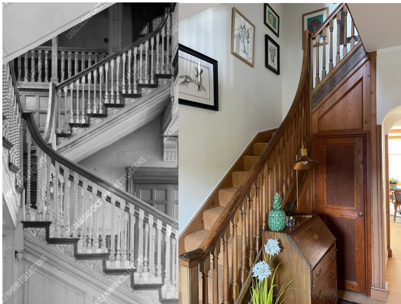
Fig 9. The open string staircase at Bryn-y-Pys hall, and the similar, but much restrained closed string staircase at The Lodge.
