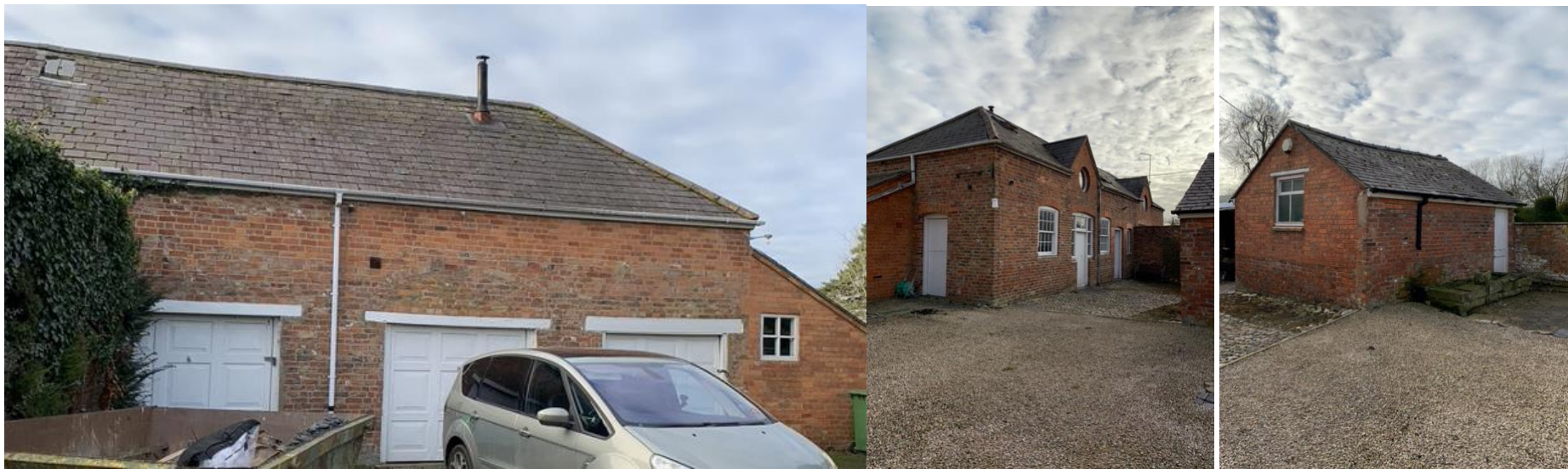
Fig 7. The stables, now divided with the neighbouring property, and a much-altered potting shed.
