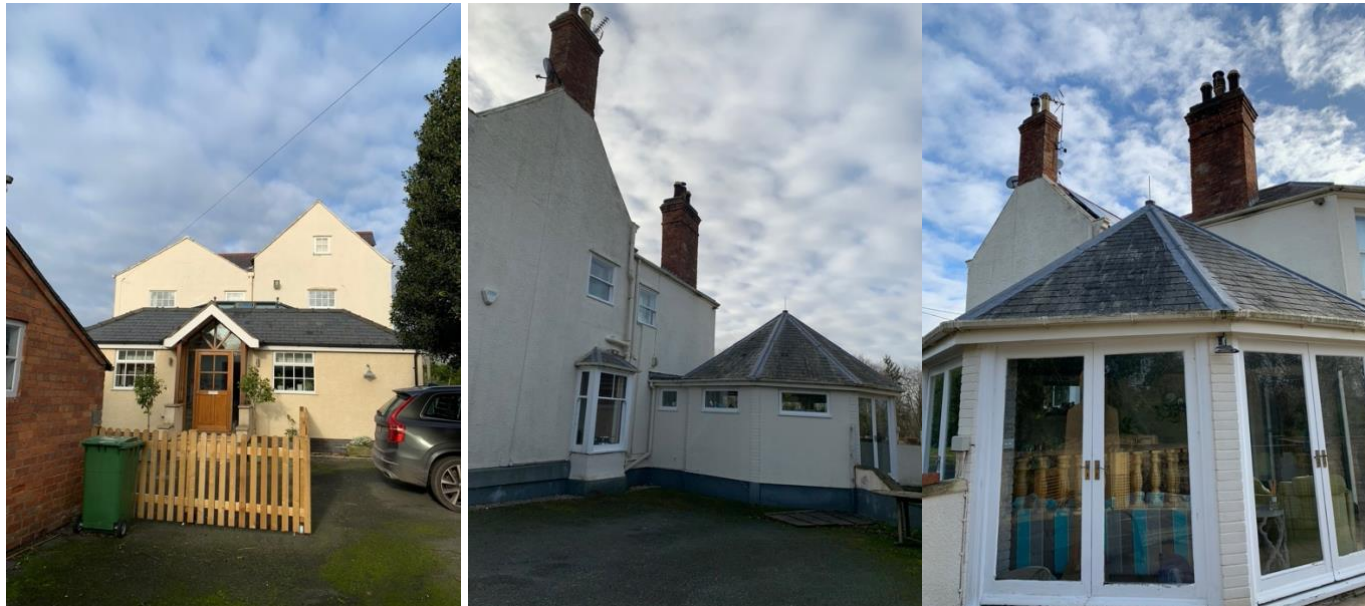
Fig 14. The modern kitchen to the southern end gable following the demolition of the original, and single storey extensions.
