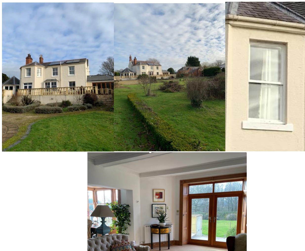
Fig 12. The rear wing at The Lodge, with an early sash window of c1840. Internally the architraves, panelling, and plastered ceiling suggests a date of the mid 18 th century, but the architraves may possibly have been remade.
