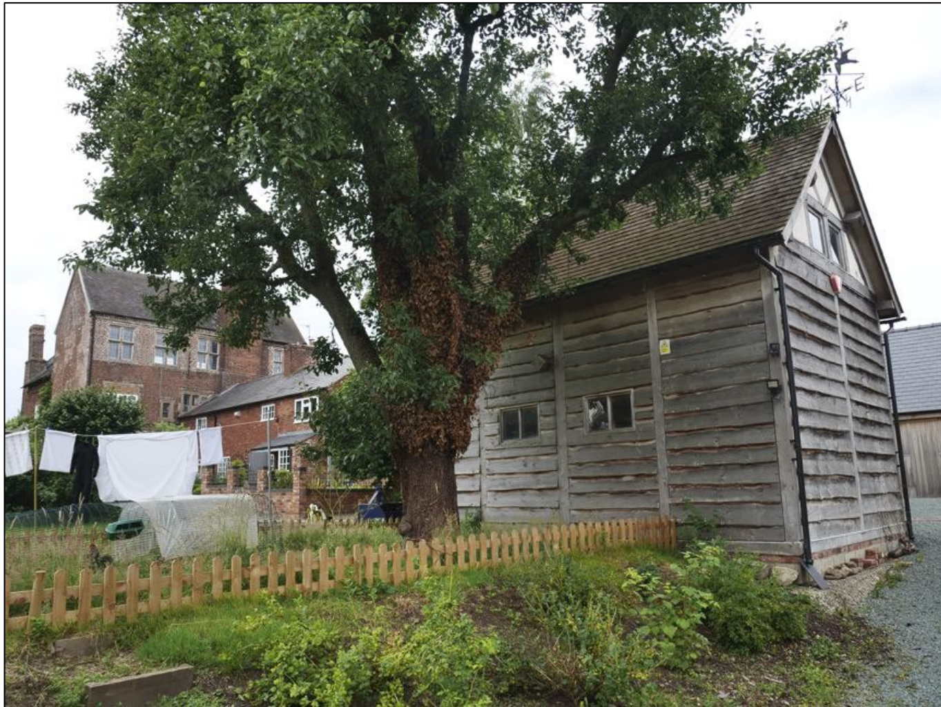
Figure 16: View of Outbuilding 3 from South East
