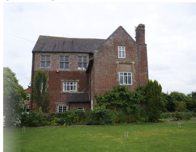
Figure 1: Existing South Side Elevation View
