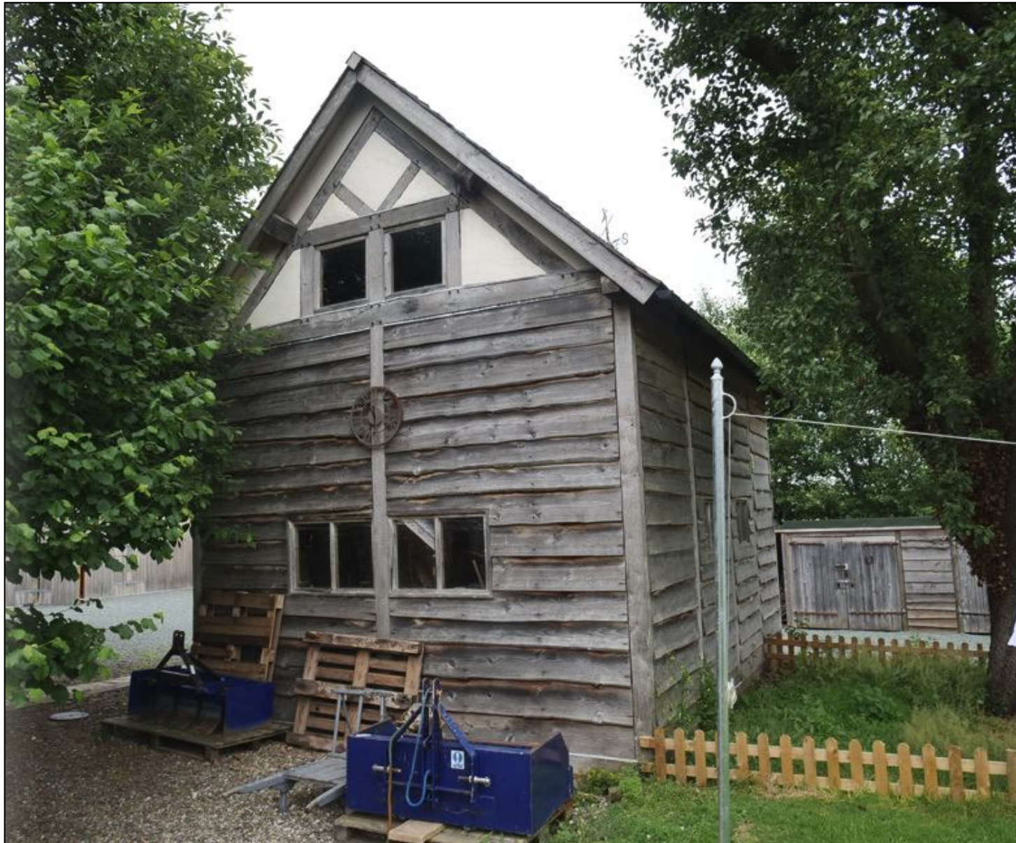
Figure 15: Outbuilding 3 Western Gable
