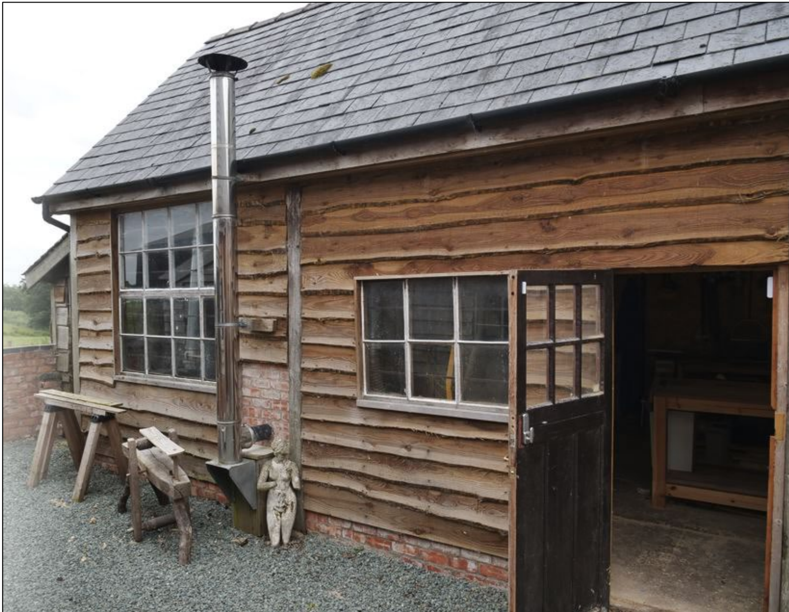
Figure 19: View of Outbuilding 2 Northern Elevation
