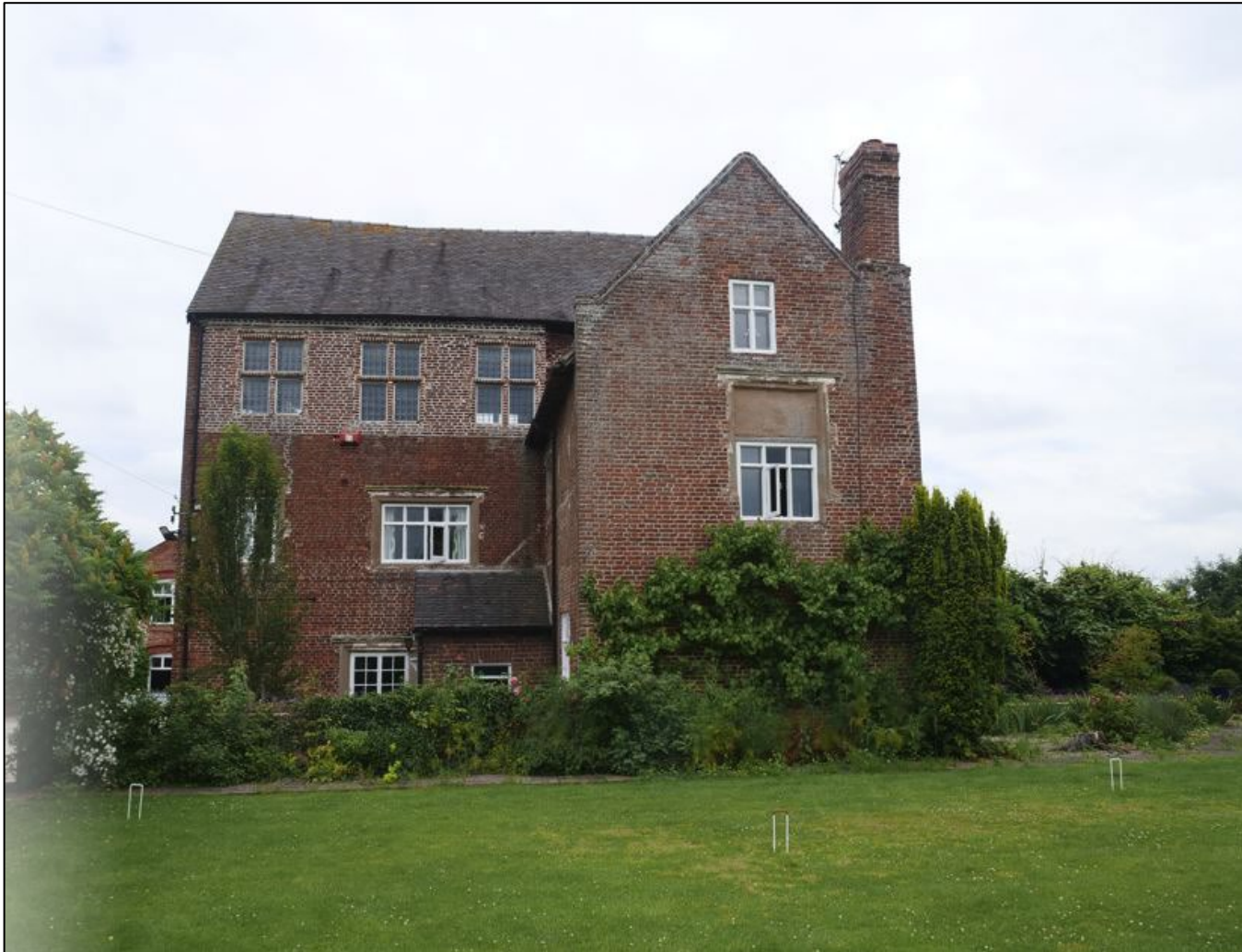
Figure 7: View of South Elevation of Main Hall
