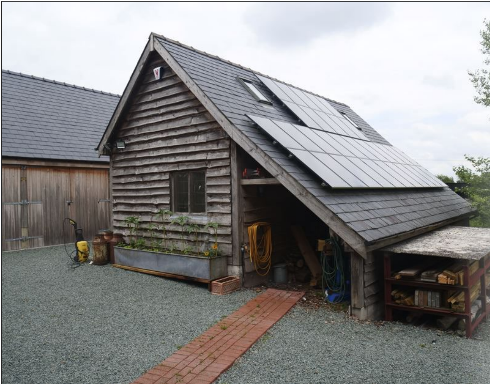
Figure 18: View of Outbuilding 2 Western Gable
