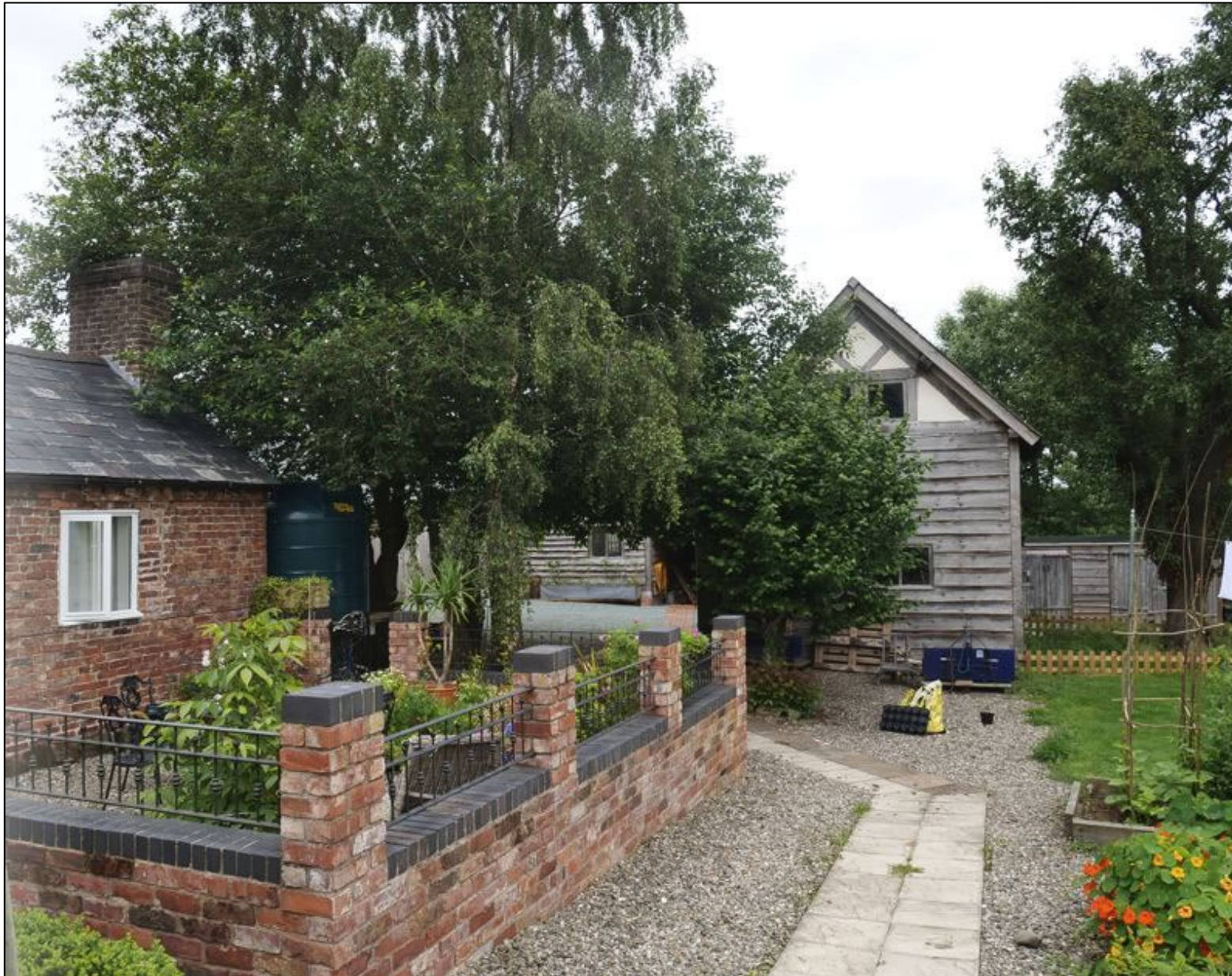
Figure 14: View of Outbuilding 3 as seen from Kitchen Path
