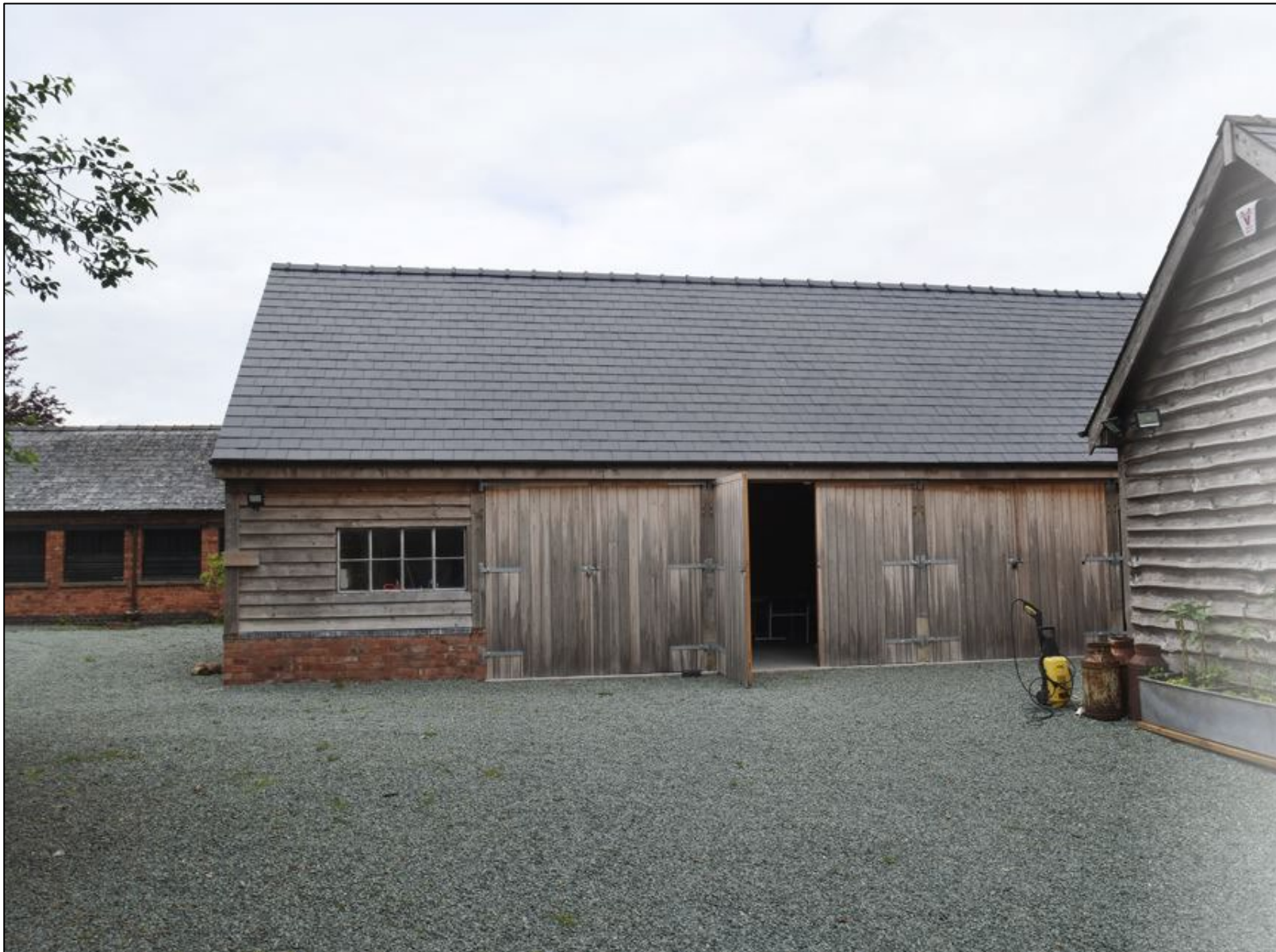
Figure 20: View of Outbuilding 1 Southern Elevation and Outbuilding 2 to right
