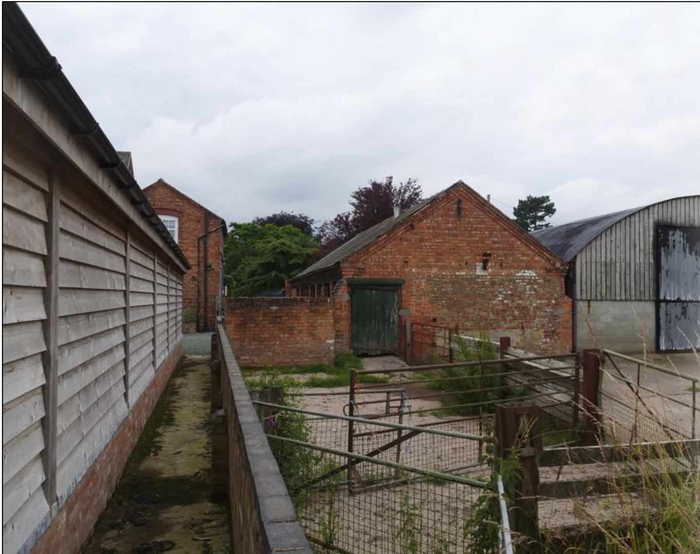
Figure 23: View of Northern Elevation of Outbuilding 1 and Neighbour's adjacent farm buildings
