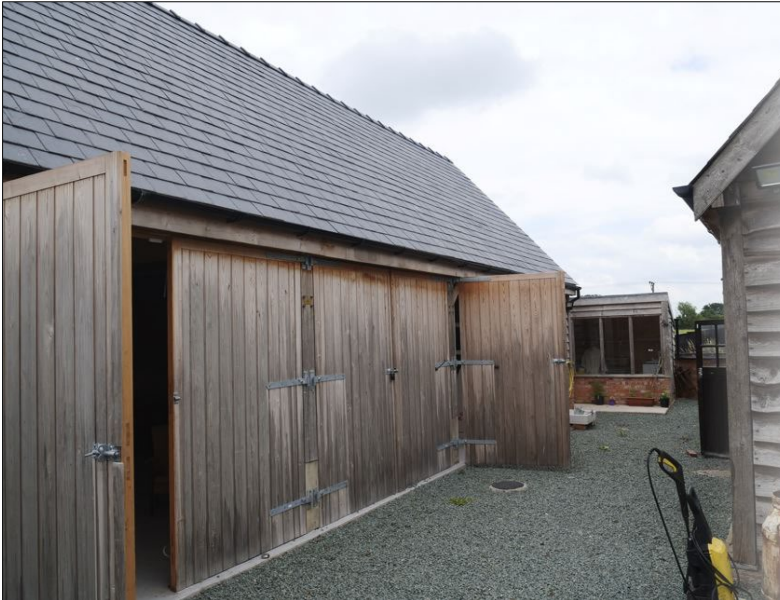
Figure 21: View of Outbuilding 1 Southern Elevation
