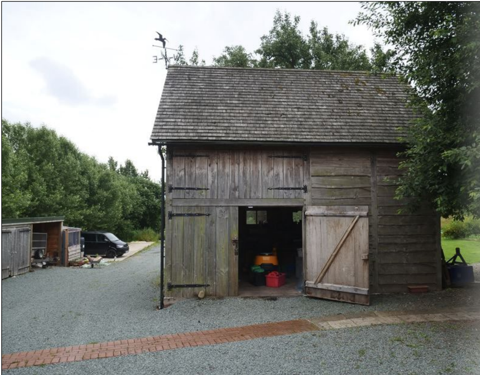
Figure 17: View of Outbuilding 3 Frontage – Northern Elevation
