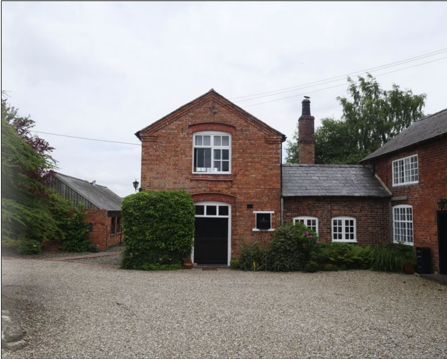
Figure 11: View of North East Wing (Outbuildings not visible behind)
