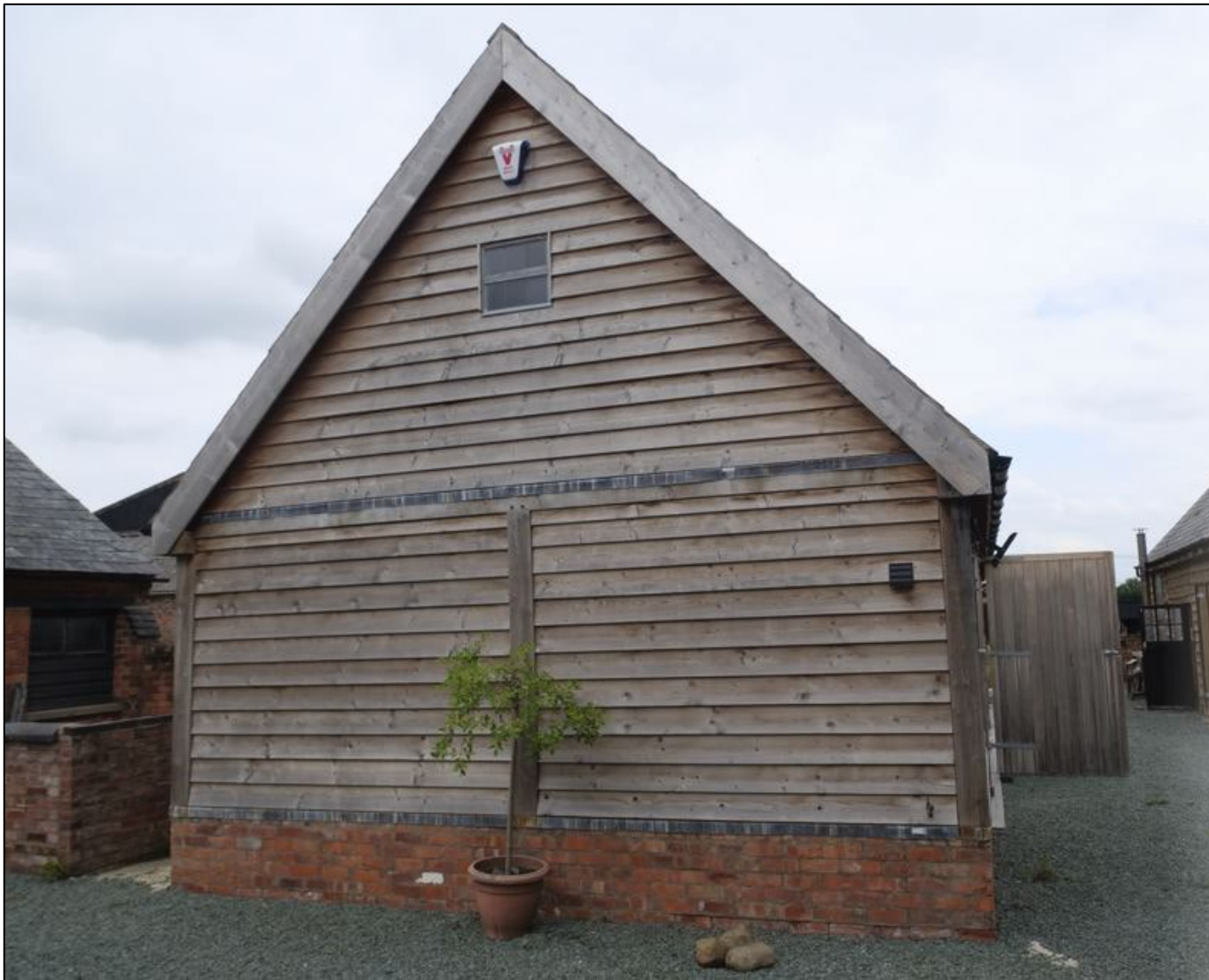
Figure 24: View of Western Gable of Outbuilding 1
