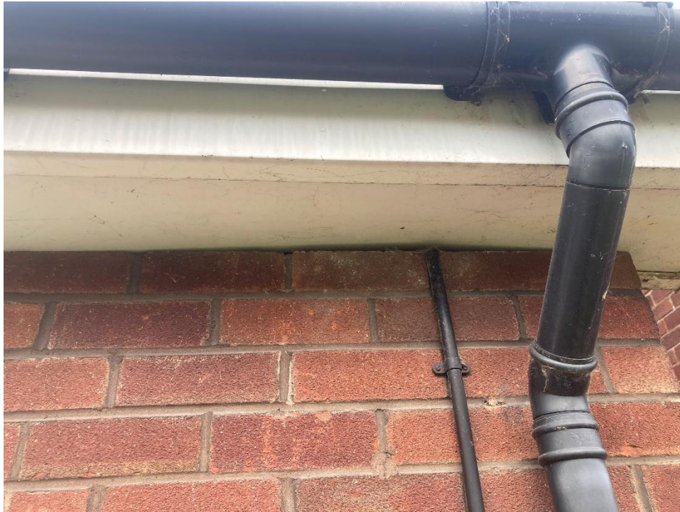
A1.6 Plate 6 – Shows well sealed soffit box and wall plate
