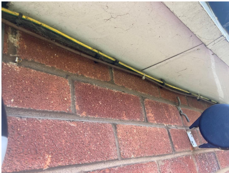
A1.6 Plate 6 – Shows well sealed soffit box and wall plate
