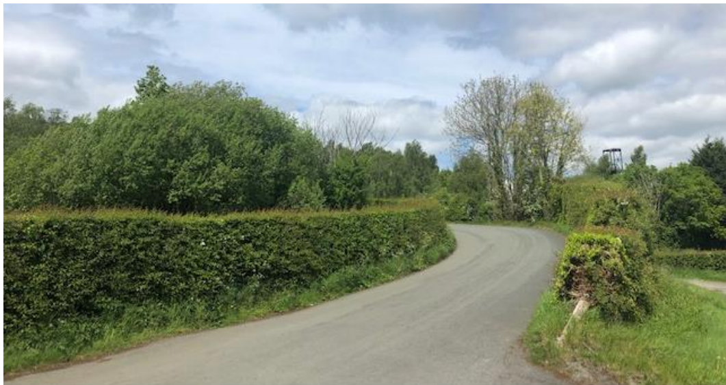
Figure 14: View from Colliery Road of the Bersham Colliery tip (visible beyond immediate tree cover and forming skyline on the left) and the winding gear protruding above the trees on the right
