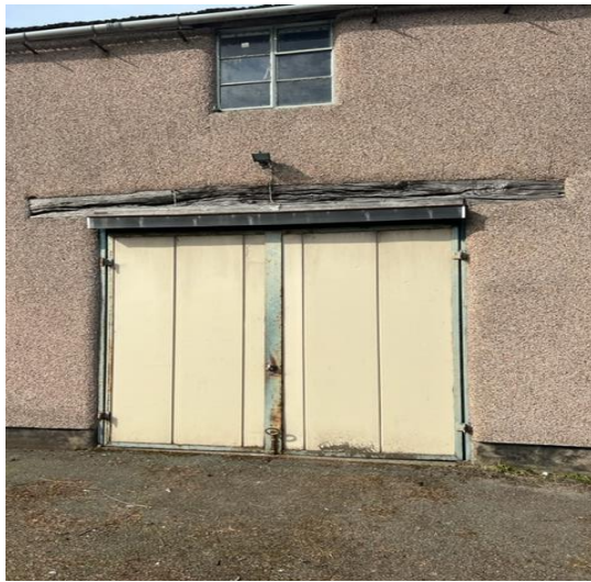
(existing supporting beam on the East elevation)
