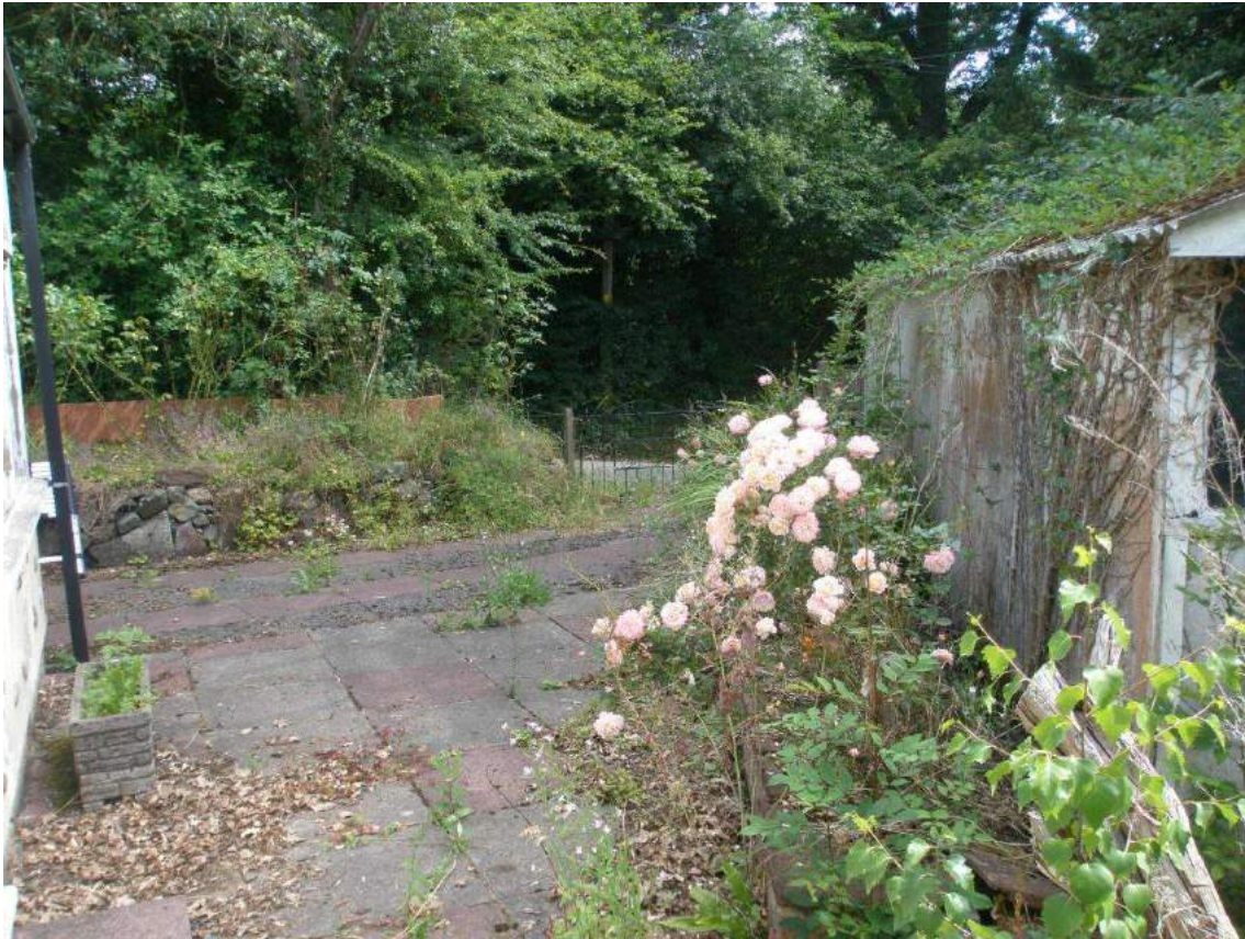
Image 6: hardstanding looking north-east towards Tower Hill, with dilapidated to right and main structure to left.
