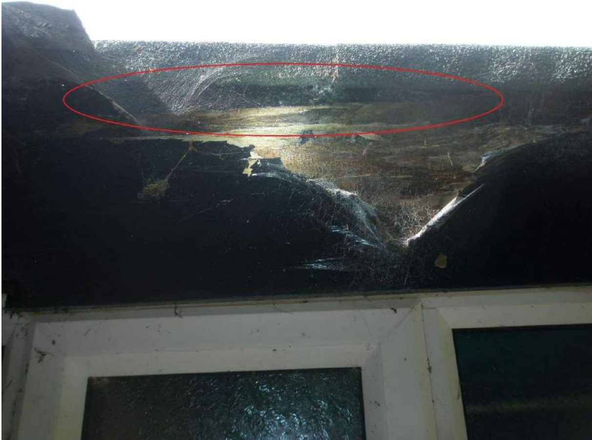
Image 12: Feature 4 as shown in Appendix C, showing top of brickwork adjacent to soffit where guttering ends with cobwebs present.
