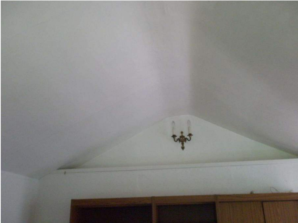
Image 8: general view of internal roof structure indicating no void present.
