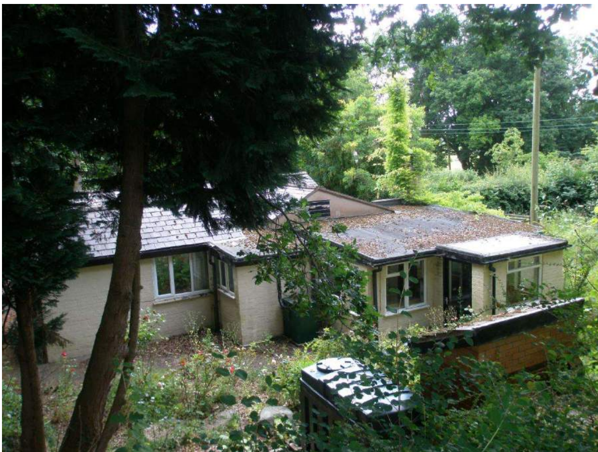
Image 3: view from steep embankment to north-west looking south-east over main structure.
