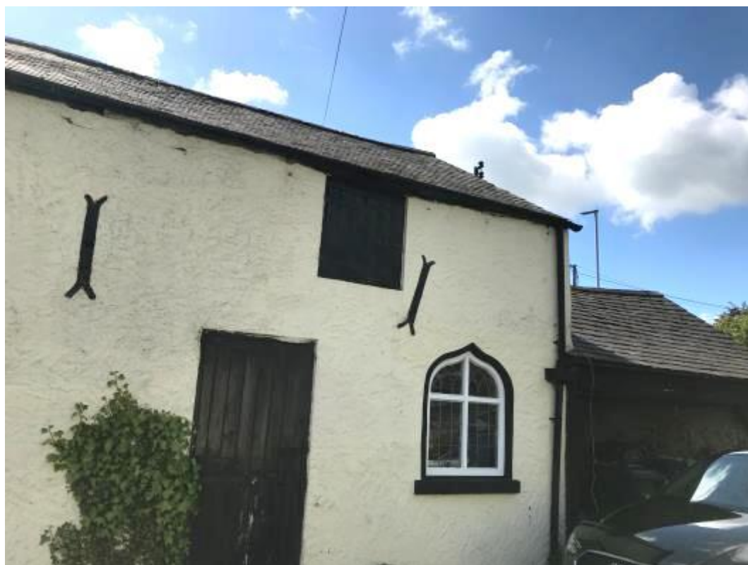
Plate 2 – Viewed from the west with the garage section visible
