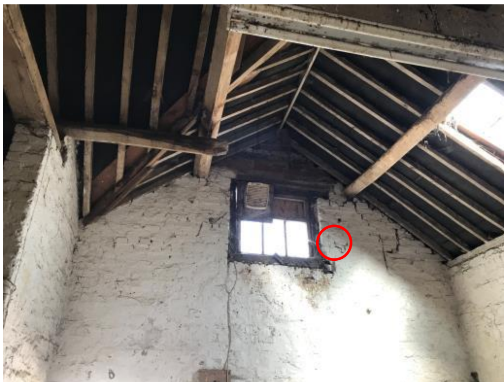
Plate 8 – Internal character of the barn displaying bitumen 1F underfelt and skylights
