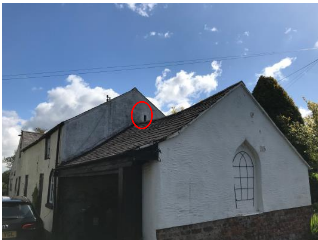
Plate 3 – Viewed from the south, with window ingress point visible
