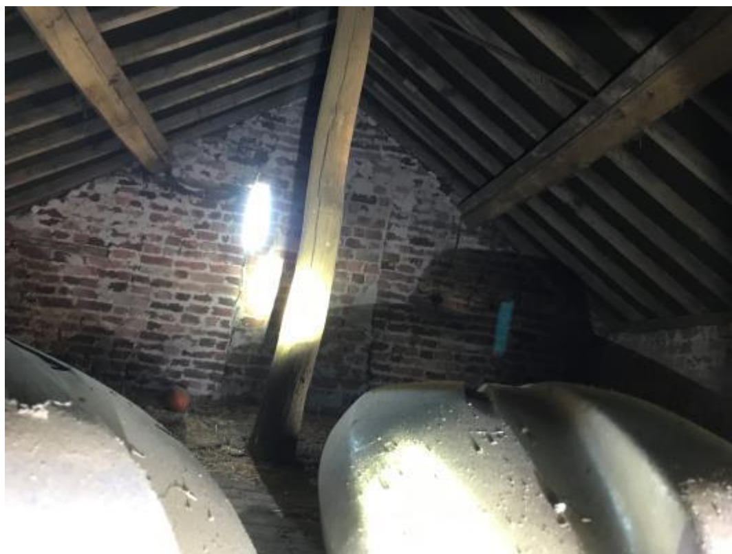
Plate 10 – Internal character of the mezzanine/first floor room
