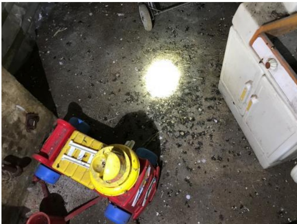
Plate 13 – Faecal splashing and nesting material
