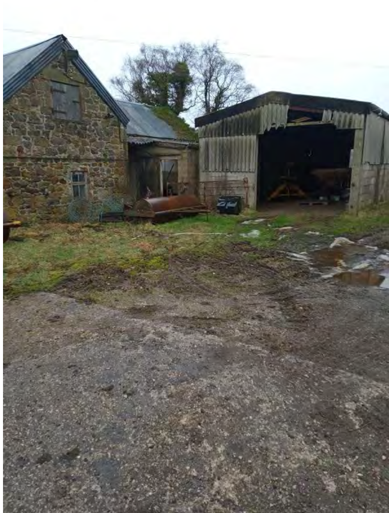
Photo 7: Yard area in the north east of the Site.
