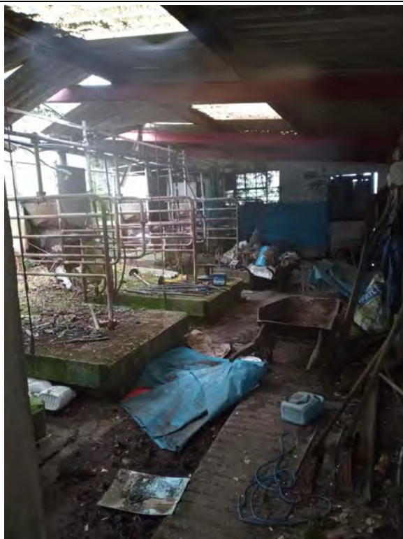
Photo 4: View with the former milking parlour in the west of the Site.
