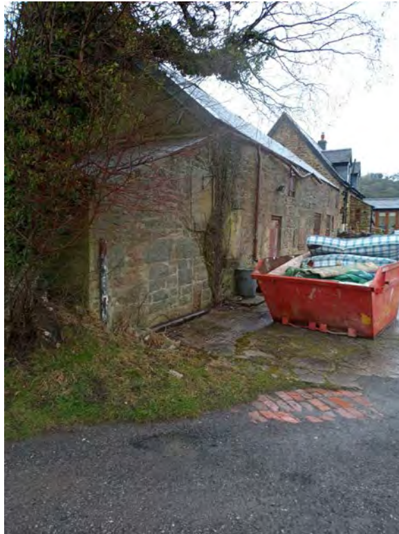
Photo 1: View across the south of the Site.
