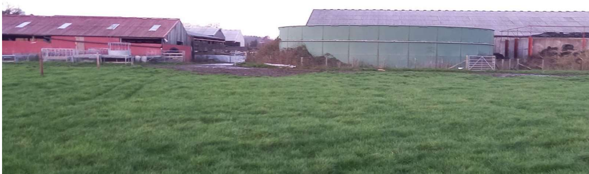
The area the proposed store will be located, adjacent to the existing store.
