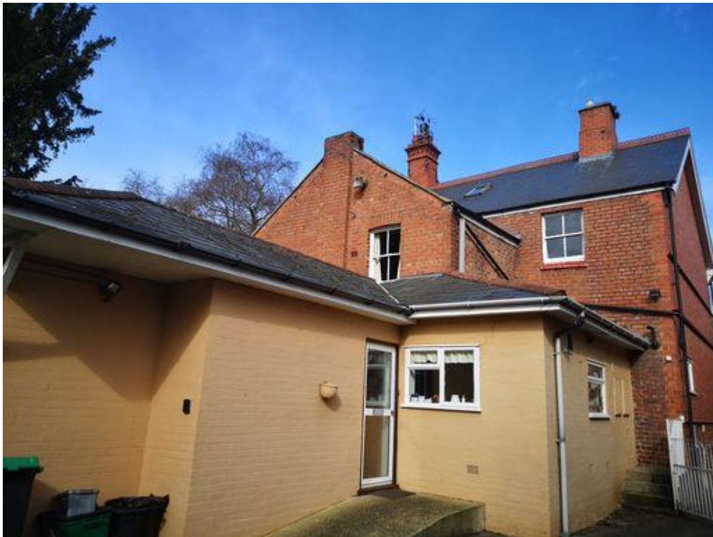
Plate 8 -Southern elevation featuring hipped roofed extensions.
