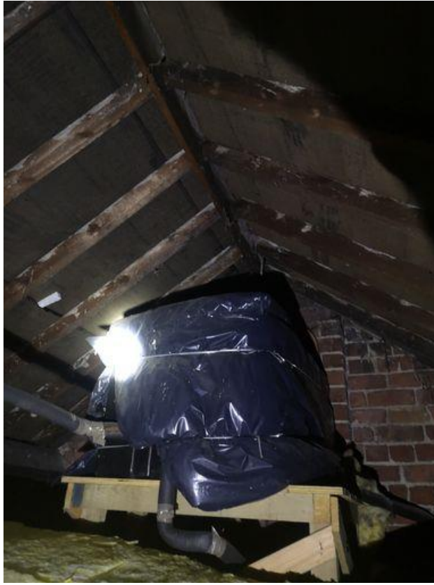
Plate 8 – internal Character of Loft 1
