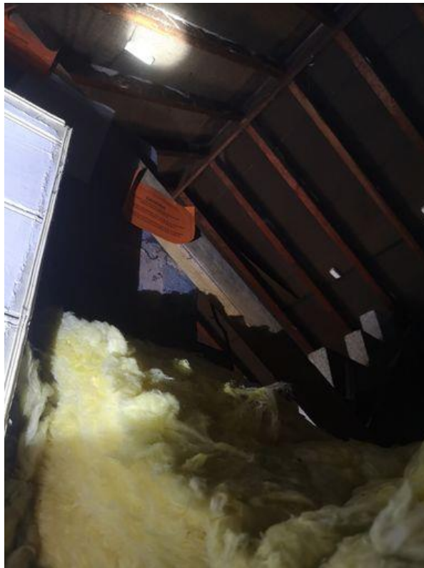
Plate 10 - Internal character of Loft 2
