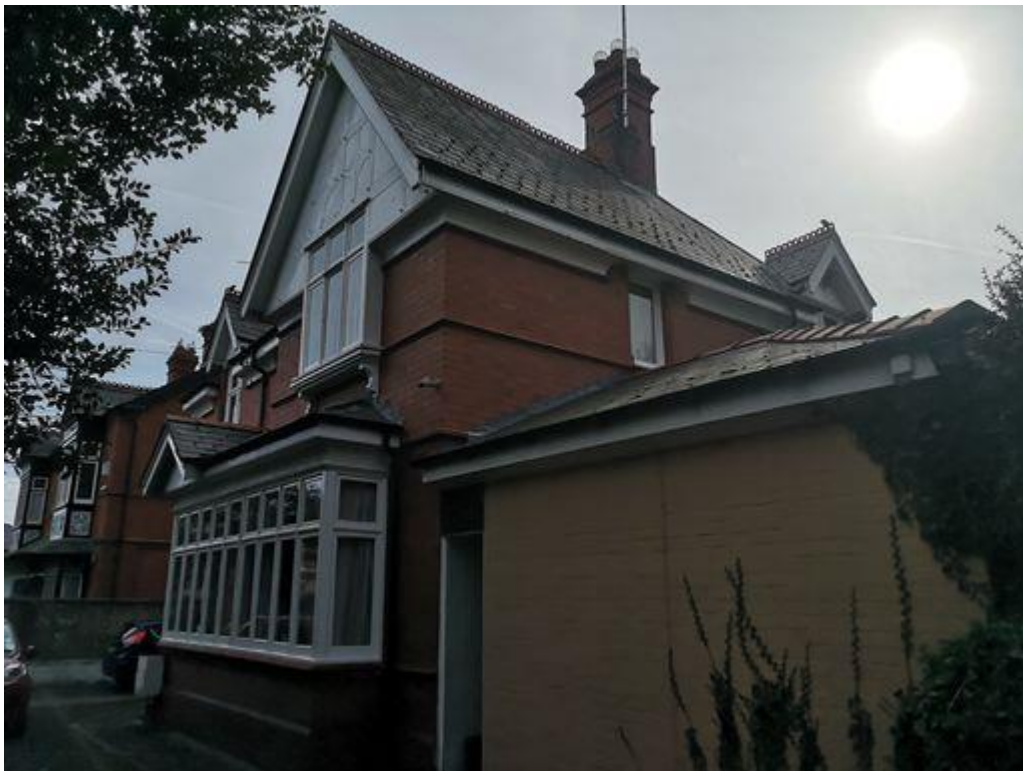
Plate 6 – Northern elevation of No.2 Belgrave Road
