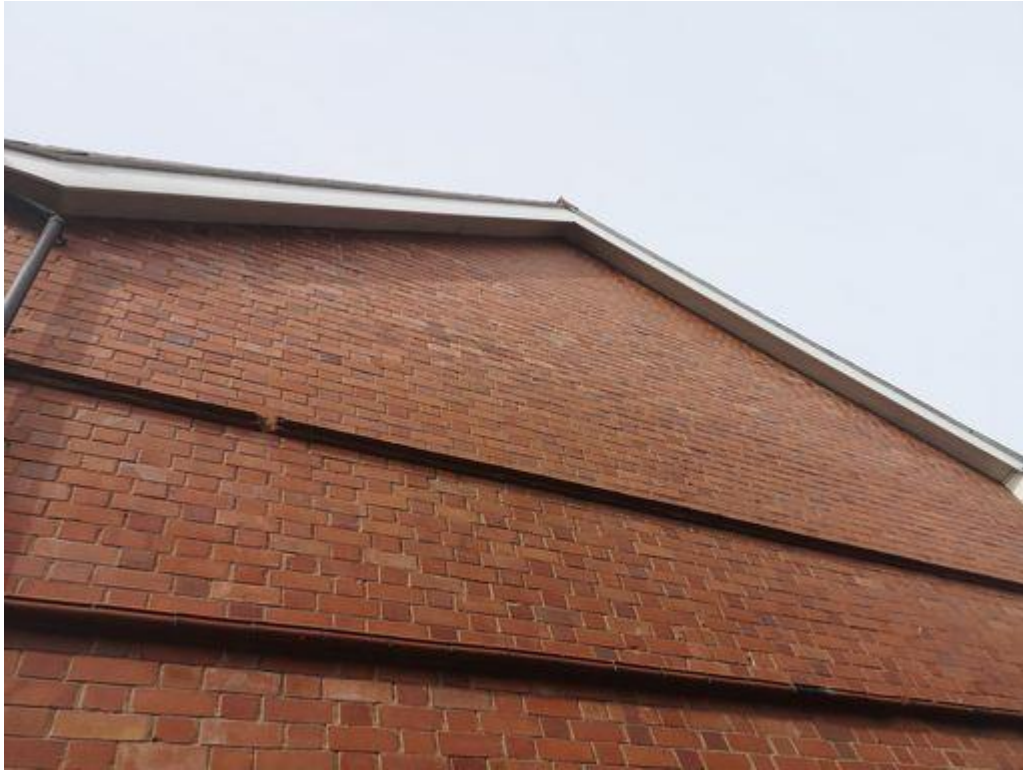
Plate 7 – Eastern gable elevation of No. 2 Belgrave Road
