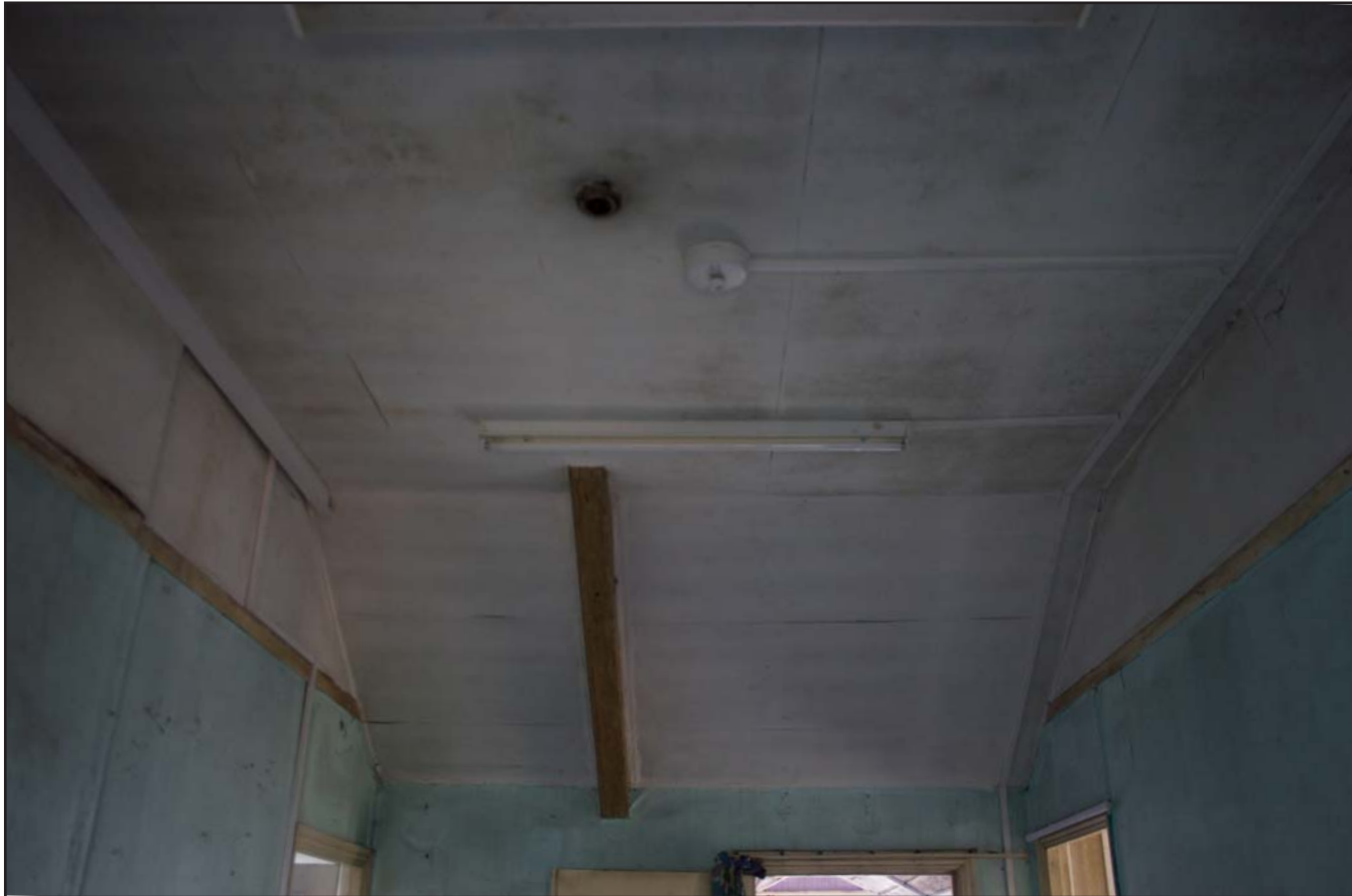
Plate 16: Living Room showing ceiling, from the southeast.
