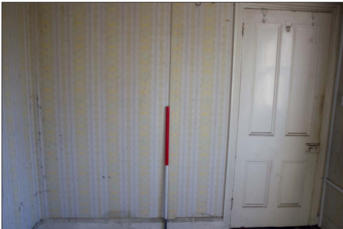
Plate 22: Bedroom 2, from the southwest. Scale 1.0m.
