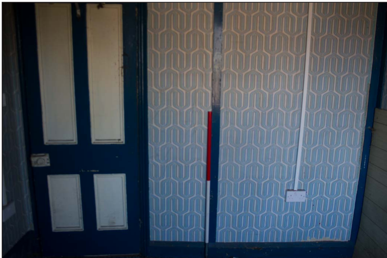
Plate 19: Bedroom 1, from the southwest. Scale 1.0m.
