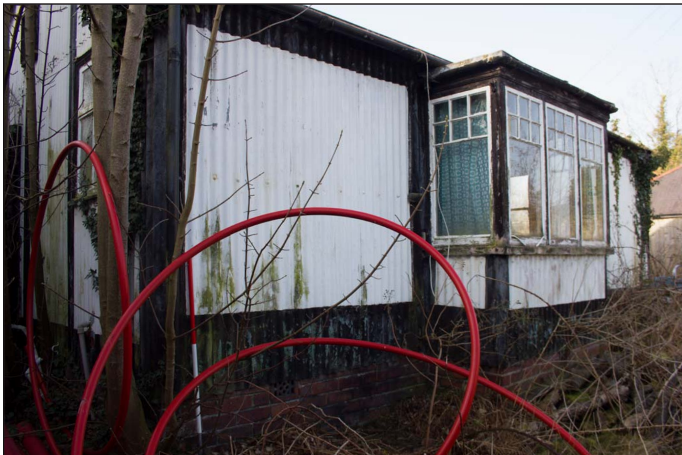
Plate 10: Northeast and northwest facing external elevations, from the north. Scale 1.0m.
