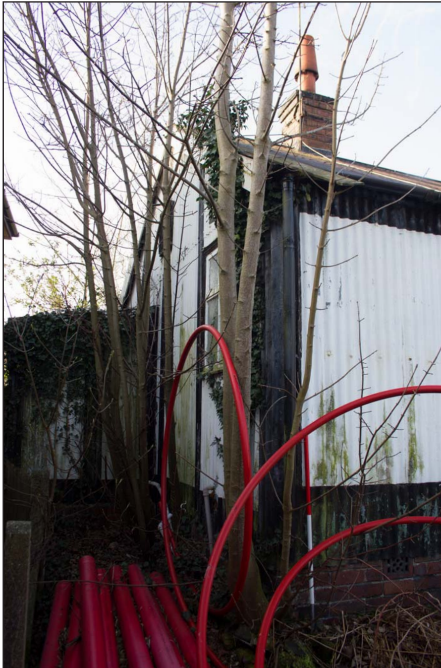
Plate 09: Northeast facing external elevation, from the north. Scale 1.0m.
