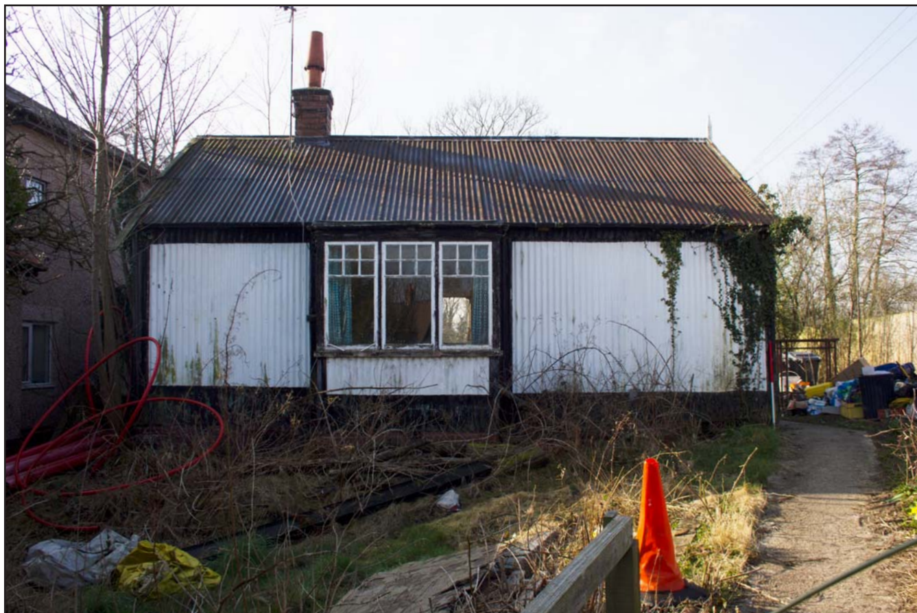
Plate 03: Northwest facing external elevation, from the northwest. Scale 1.0m.
