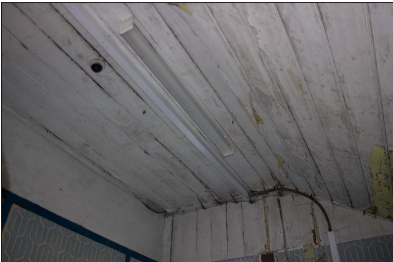
Plate 20: Bedroom 1 showing ceiling, from the north.
