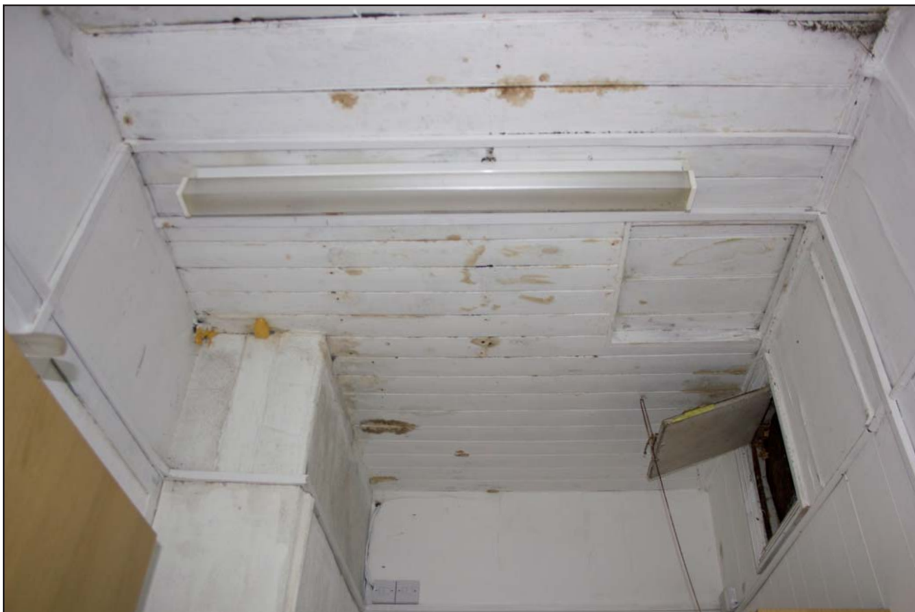
Plate 26: Kitchen showing ceiling, from the southeast.
