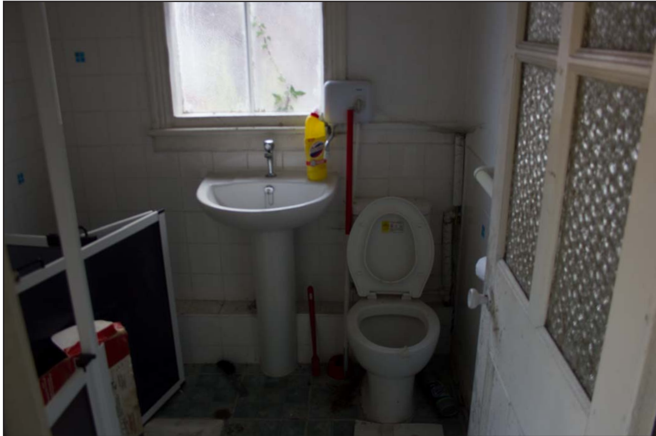
Plate 17: Bathroom, from the southwest. Scale 1.0m.
