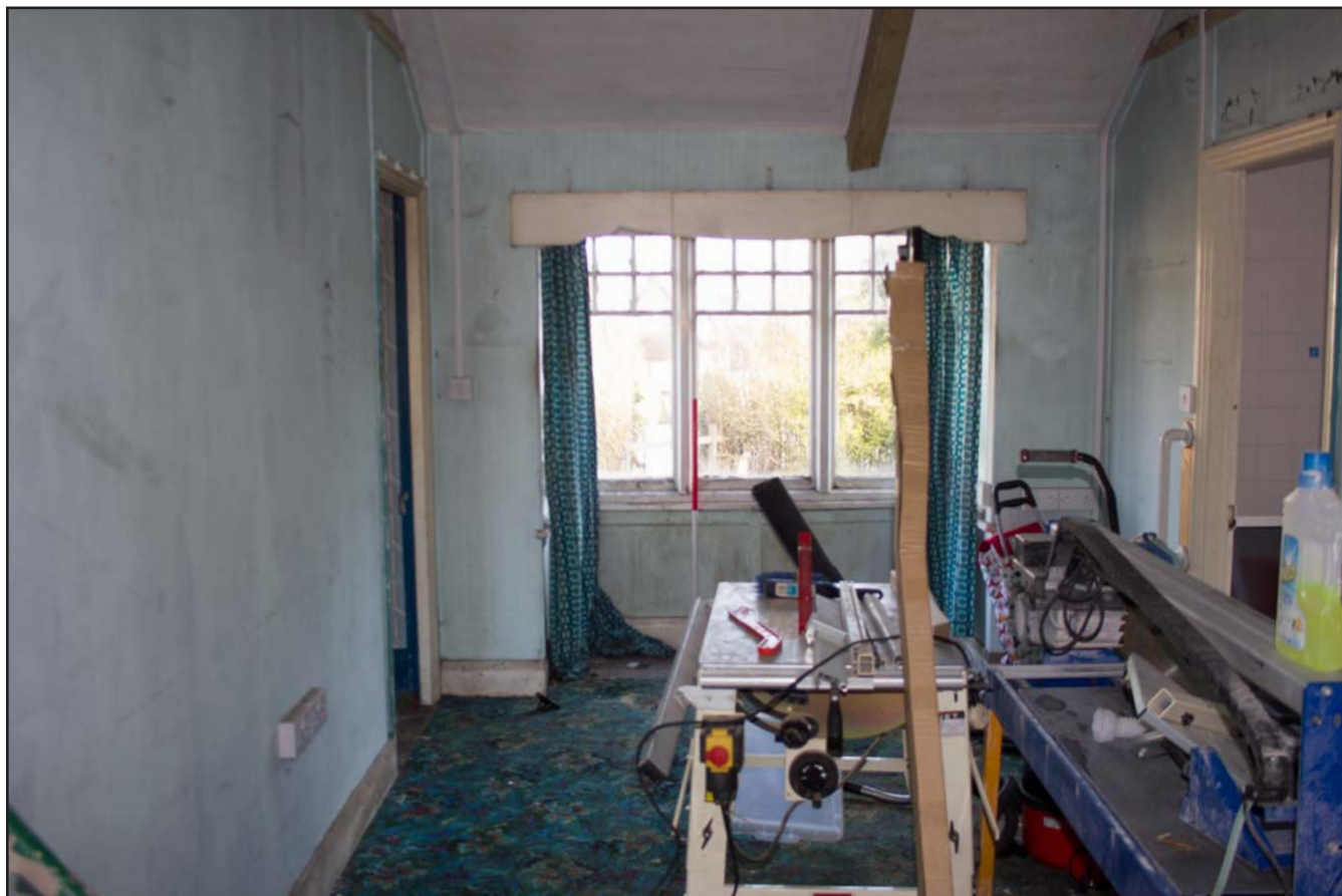
Plate 12: Living Room, from the southeast. Scale 1.0m.
