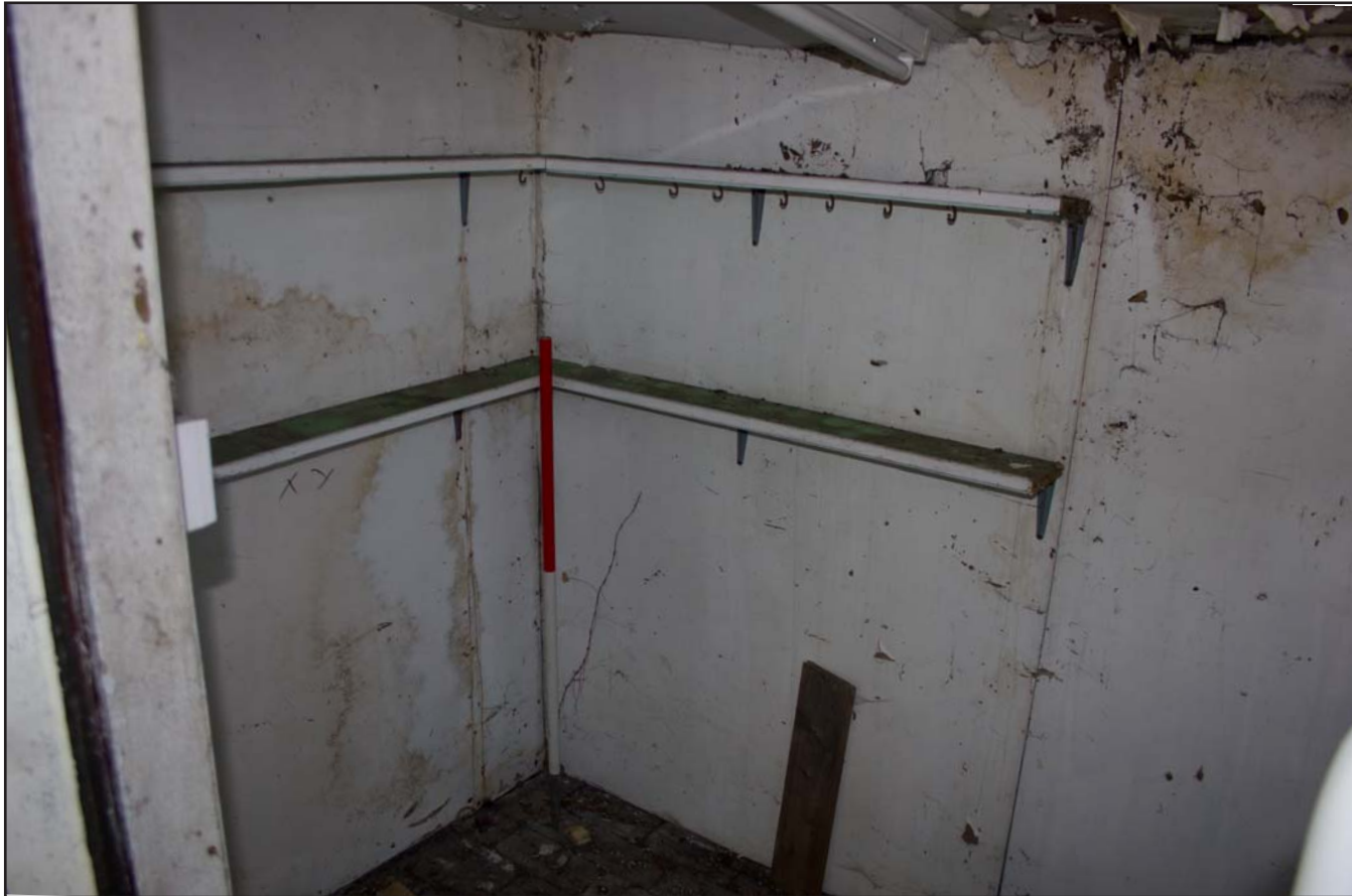
Plate 27: Lean-to outbuilding, from the south. Scale 1.0m.
