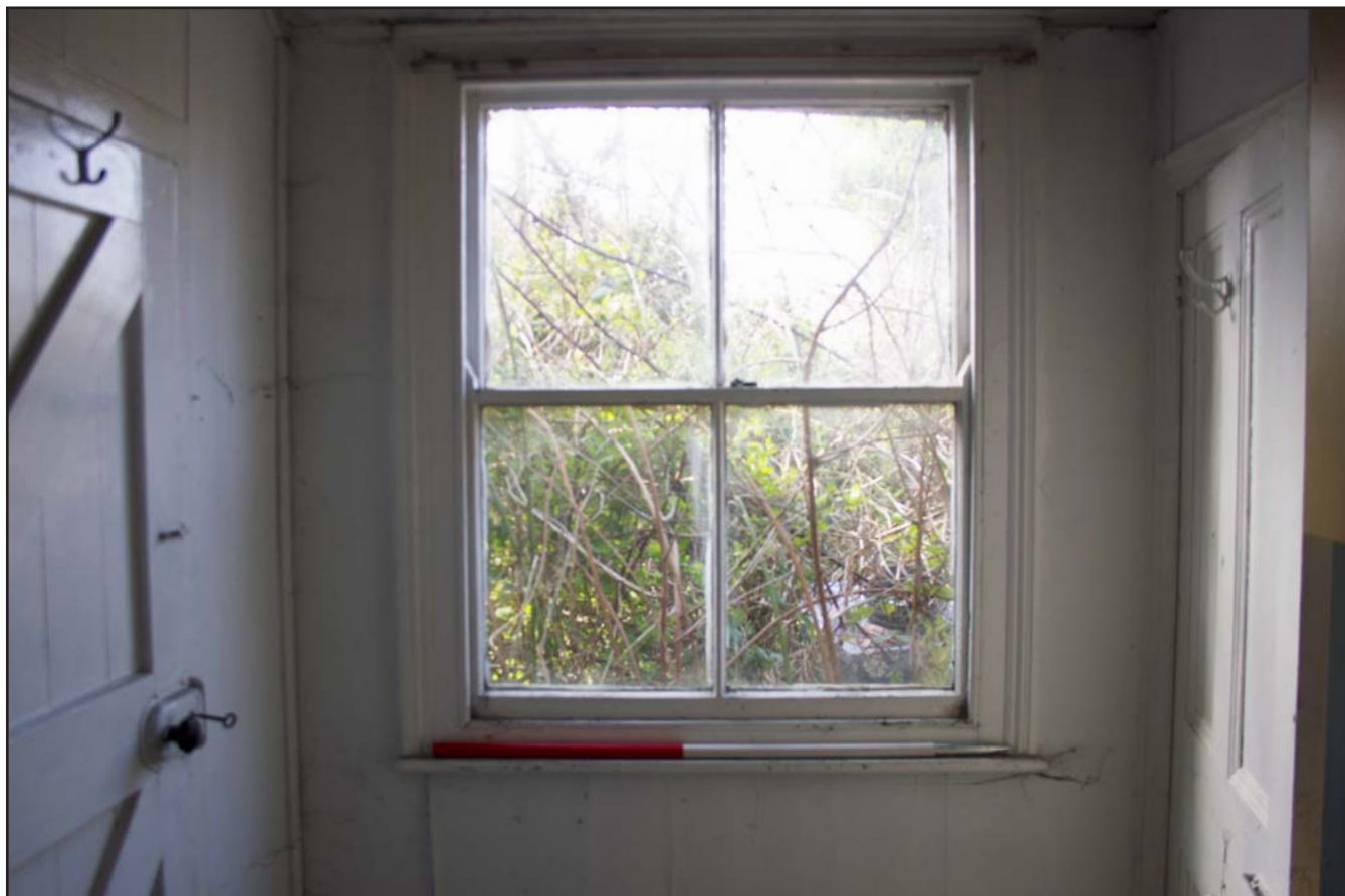
Plate 25: Kitchen, from the northwest. Scale 1.0m.
