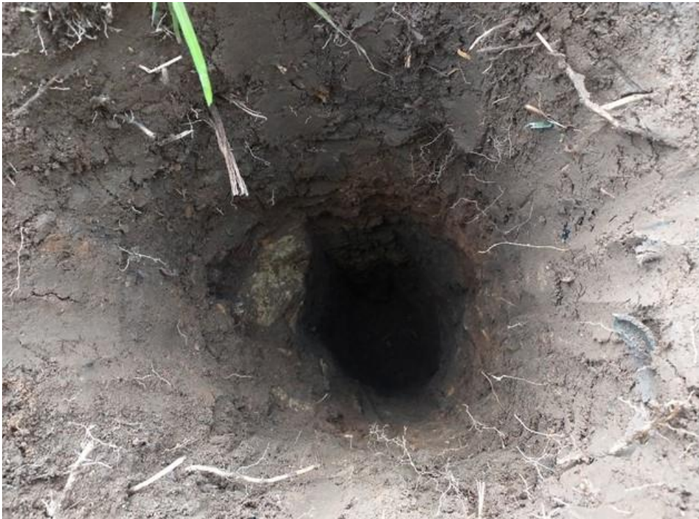
Photo 7: HP04 hand pit wall shows occasional concrete or sandstone cobbles seen in made ground between 0.09 and 0.6mbgl.
