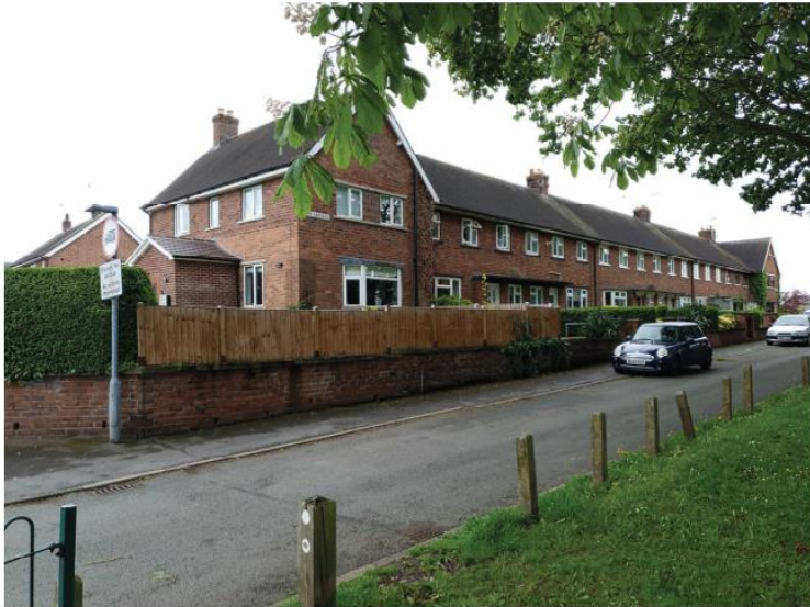
Figure 6 – Timber Boundary Fence
