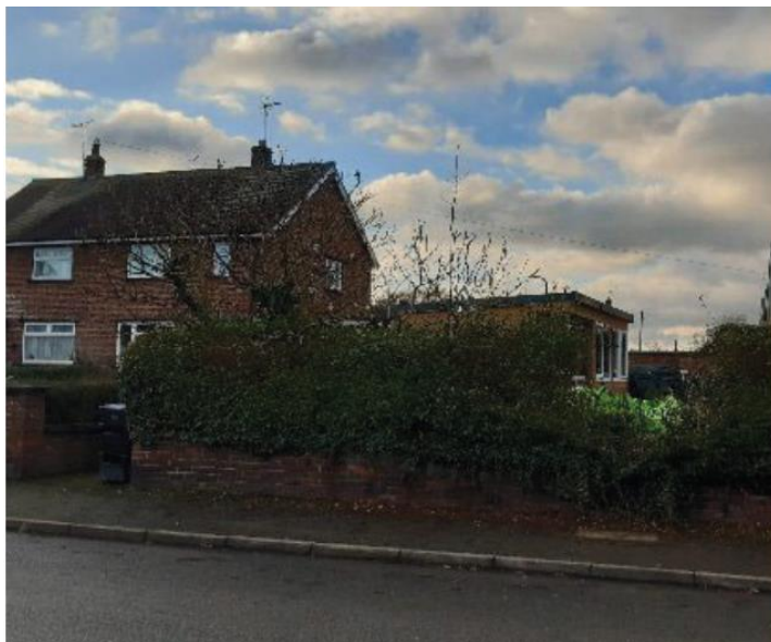
Figure 3 – outbuilding viewed from Bridge Street – the photo above demonstrates how the existing hedge shields the views of the outbuilding and a condition requiring the retention of this hedge will ensure that it continues to shield the outbuilding from view. However, even without the hedge in place the building is similar to a normal outbuilding that you would expect to see within the residential curtilage of a property.
