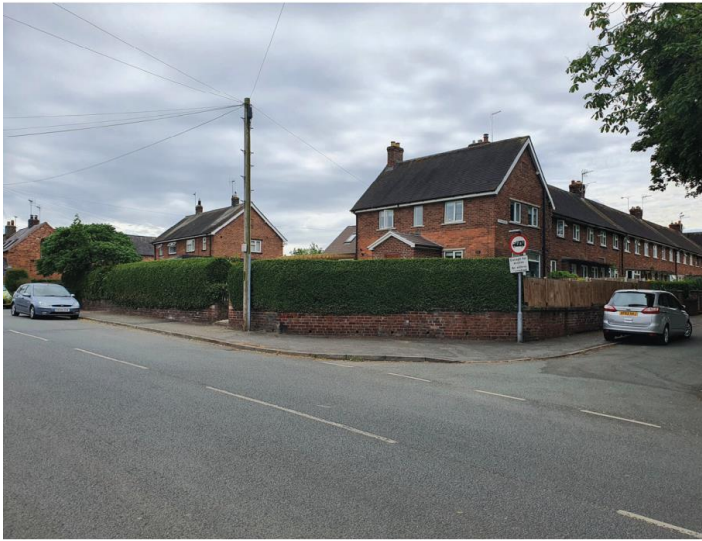
Figure 2 – Site when viewed from Bridge Street – As can be seen from the above photograph the works undertaken can barely be seen from the street scene and therefore do not have a detrimental impact upon the character and appearance of the area or the Conservation Area.
