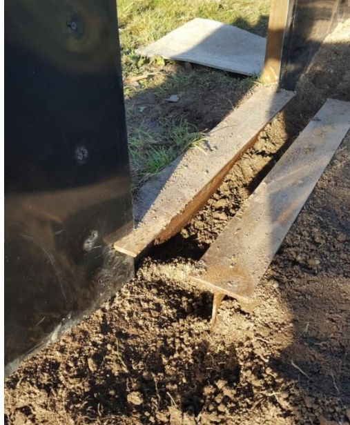
Figure 3.3. RSJ site entrance, with suitable excavations
