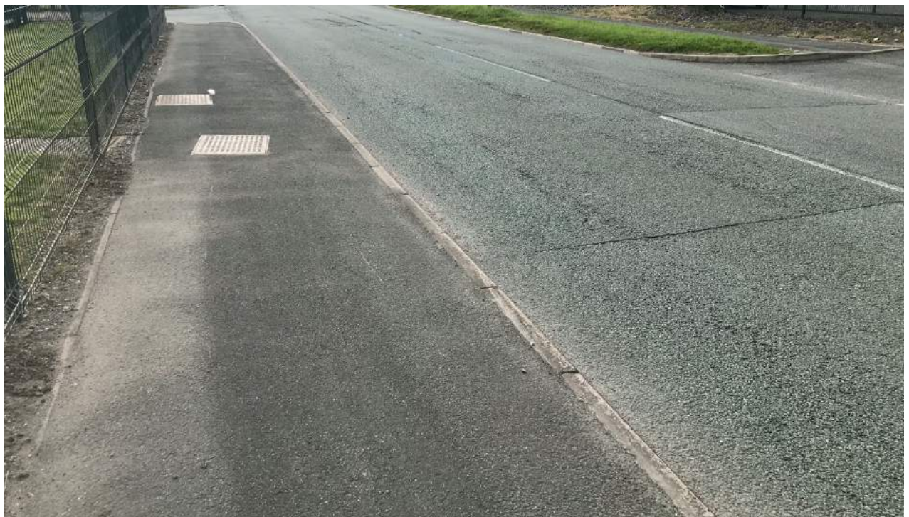
Photograph 2.4 : Coed Aben Road – Carriageway and Footway
