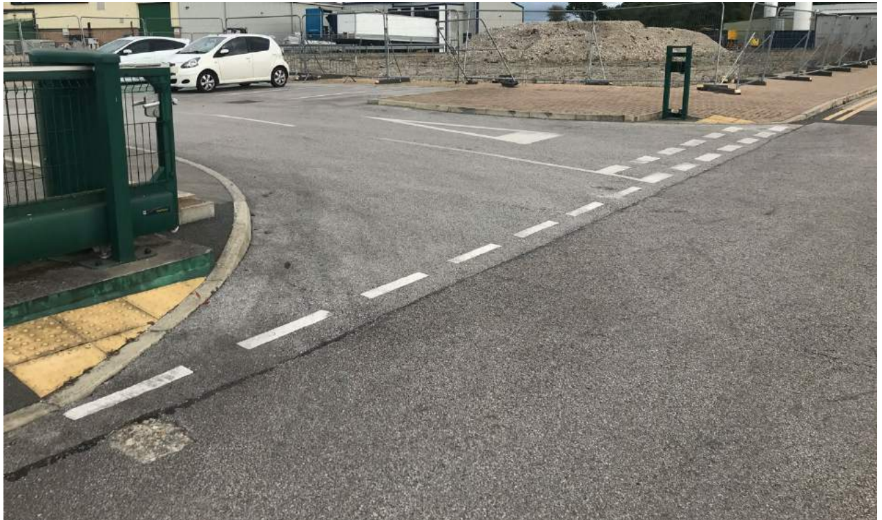
Photograph 2.3 : Internal Car Park Access
