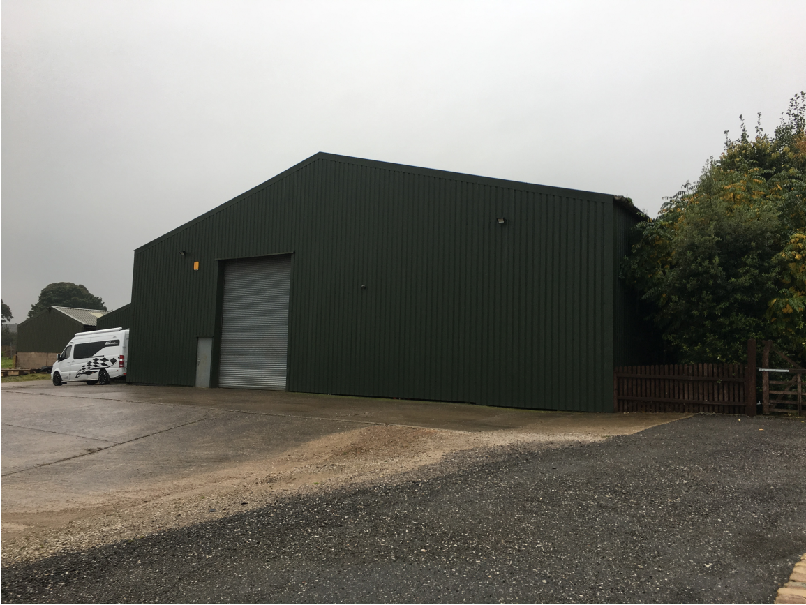
PHOTOGRAPH 2: EAST ELEVATION (VIEWED FROM NORTH-EAST) OF FORMER OUTBUILDING PREVIOUSLY GRANTED CONSENT TO BE REMOVED AS PART OF PLANNING APPLICATION (P/2016/0409)
