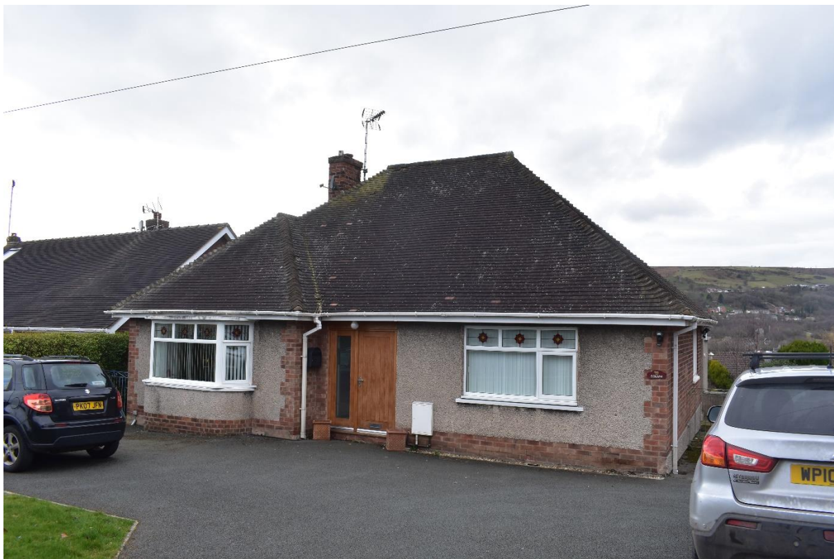
Figure 3.2: The front (east-facing) aspect of the dwelling.
