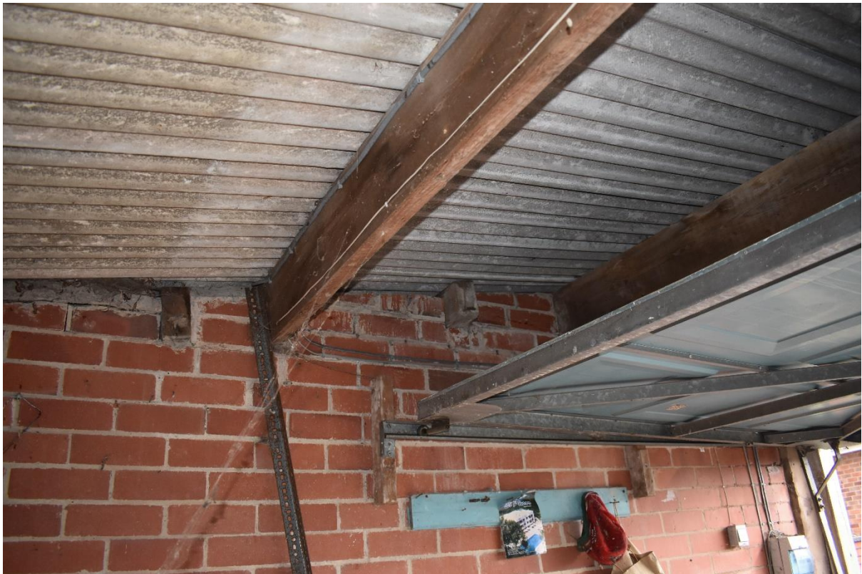
Figure 3.12: The wooden supports and roof-wall join of the interior of the outbuilding to be removed.
