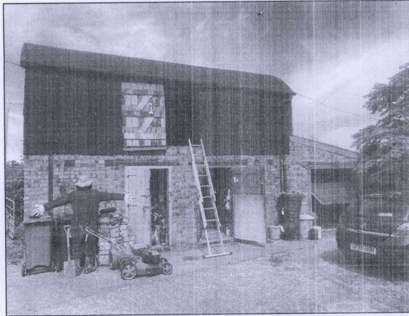
A1.1 Plate 1: View on eastern aspect of building
