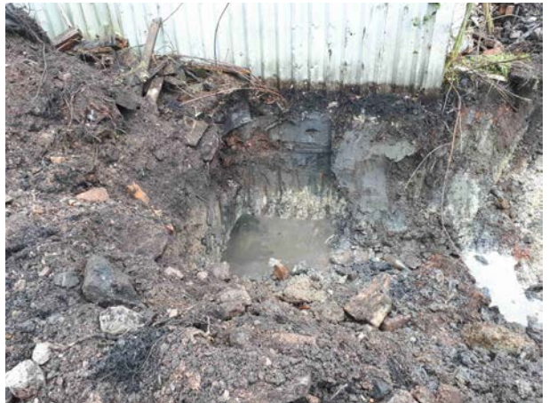
12.04.18 – Excavation along the old water pipeline northwards adjacent to the tin shed.
