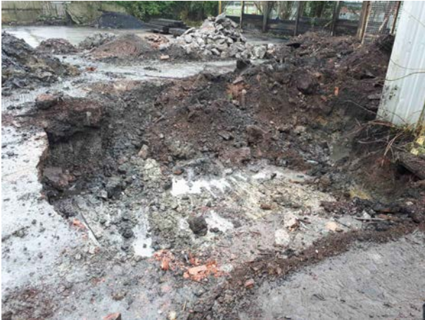
12.04.18 – All diesel impacted made ground segregated from the excavation.
