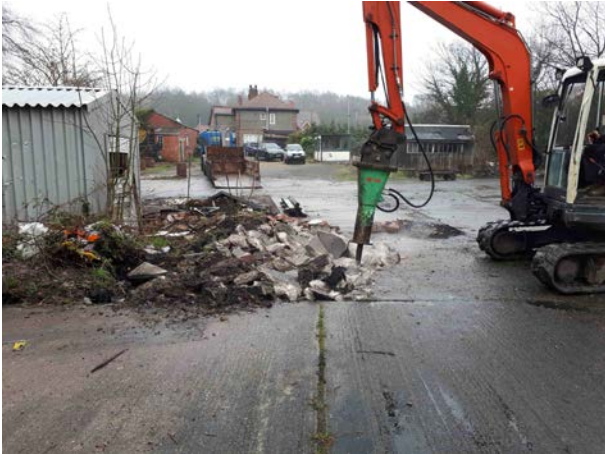
12.04.18 – Breaking out of concrete hardstanding in a 2m radius around TP4.
