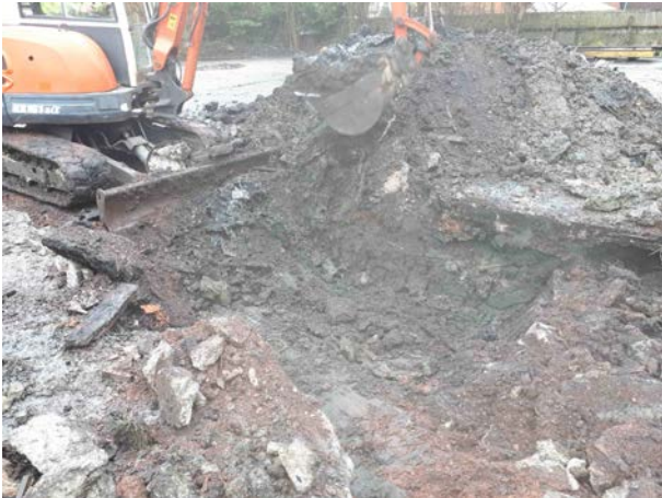
12.04.18 - Excavation continues southwards along the extent of the old water pipeline.
