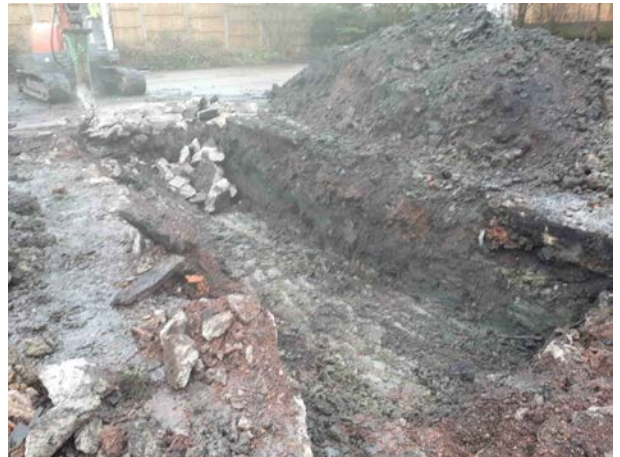
12.04.18 - Excavation undertaken to underlying natural clay, diesel impacted made ground stockpiled to the west of the excavation.
