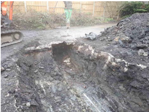
12.04.18 – Breaking out concrete to the south of the drum removed to confirm contamination has only moved northwards.
