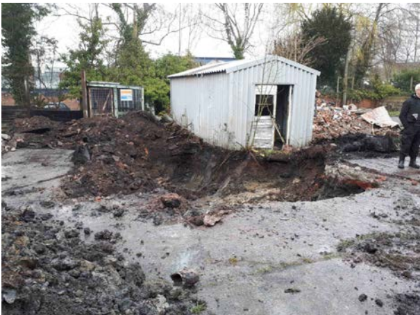
12.04.18 – Facing north towards the initial excavation.
