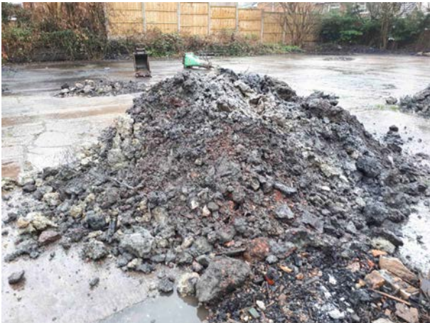
12.04.18 – Diesel impacted arising segregated and placed on concrete hardstanding surface.
