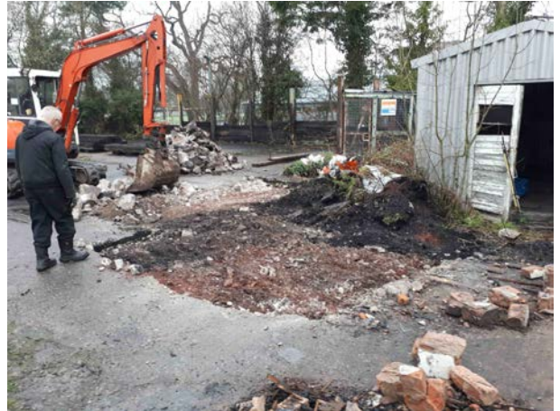
12.04.18 – Exposed made ground following the removal of concrete hardstanding, consisting of crushed brick.
