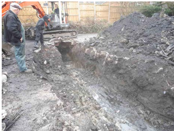
12.04.18 – Excavation continued south confirms no diesel impacted made ground to the south of the drum.
