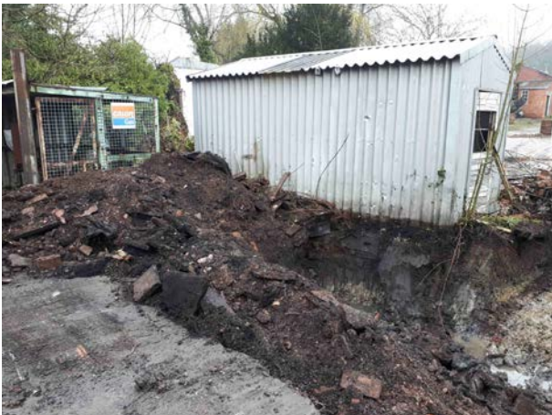
12.04.18 – Extent of northwards excavation of the pipeline to the northern boundary of the site.
