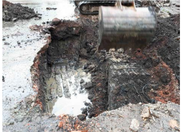
12.04.18 – Excavation of made ground identified mixed waste with diesel staining. Underlying natural clay exposed.
