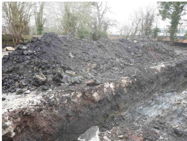
12.04.18 – Extent of impacted waste material from the excavation placed in concrete hardstanding adjacent to the excavation.
