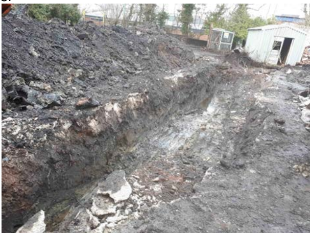
12.04.18 – Extent of excavation prior to replacement of unimpacted arisings.
