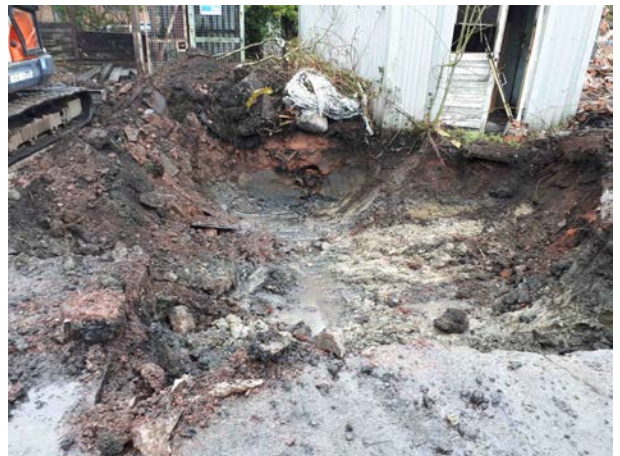
12.04.18 – Made ground excavated to natural clay, disused water pipe visible at the centre of the image.
