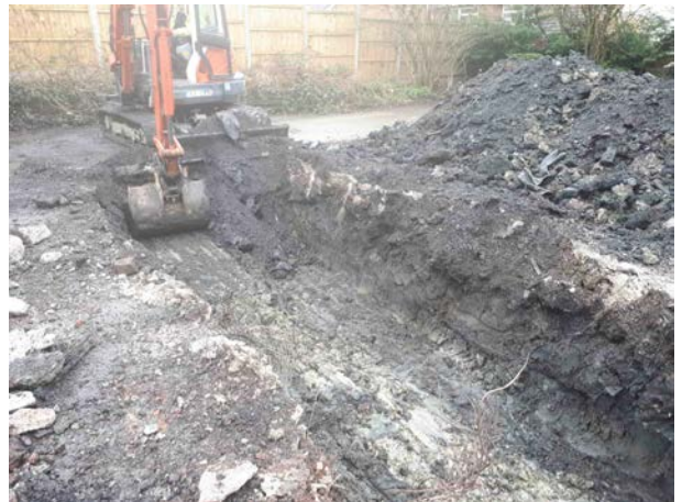
12.04.18 – Made ground being excavated to the natural clay.
