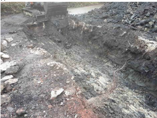
12.04.18 – The western portion of excavation continued to a greater depth as the trench continued into the underlying clay.
