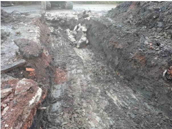
12.04.18 - Exposed clay along the central extent of the excavation continuing southwards.
