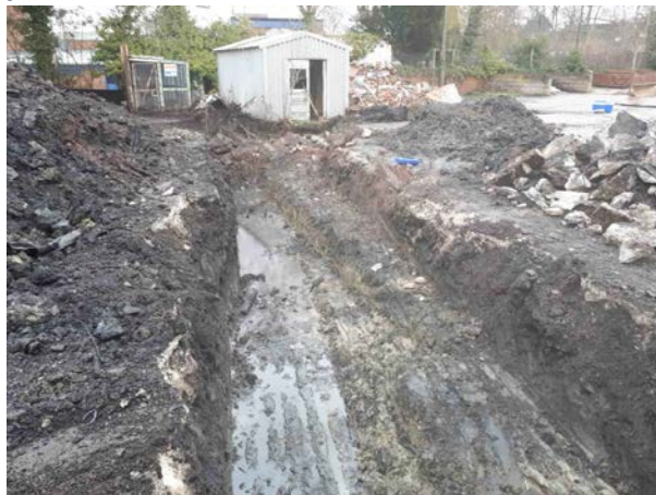
12.04.18- Facing north along the extent of the excavation with impacted material to the west and clean arisings to replace to the east.
