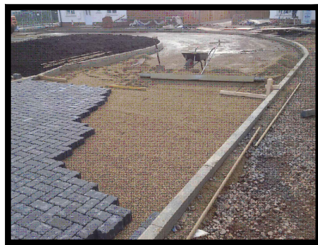
Permeable Paving (Full Infiltration)
